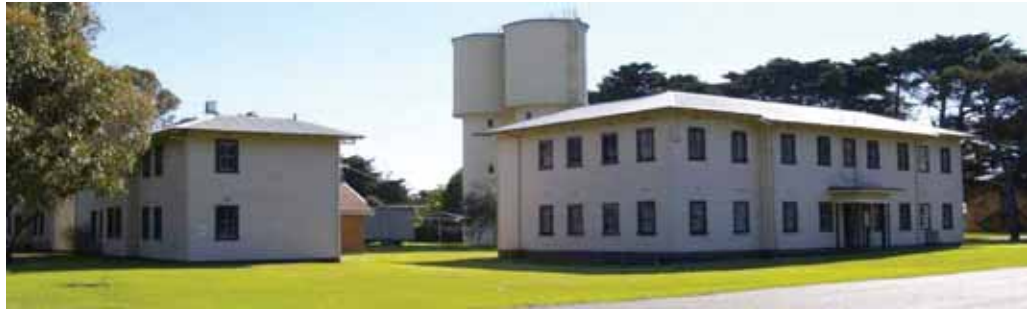
Photograph 3.19 Assets 24, 27 and Water Towers – Single Officers’ Precinct (Photograph courtesy DS-VT)
