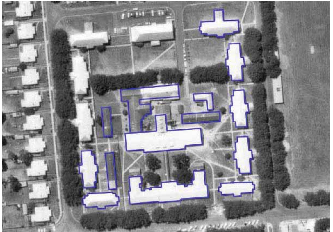
Figure E.2 Mechanic's Precinct 1967 (Courtesy RAAF Museum) – Buildings outlined have been demolished (Source: 2005 Woodhead International RAAF Williams Point Cook HMP page 21)
