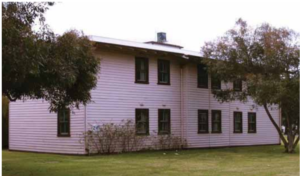
Photograph 3.18 Asset 24 – Single Officers’ Quarters (Photograph courtesy DS-VT)
