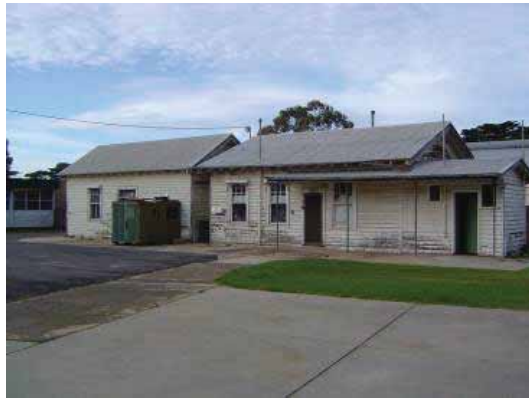
Photograph E.0.9 Former Barracks Office and Store (Woodhead International, 2004)
