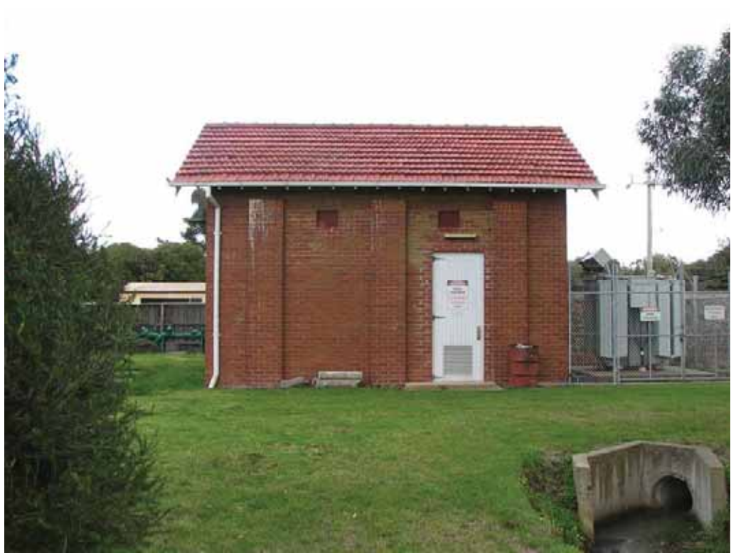
Photograph E.0.3 Building 81 - Substation (Image courtesy of DS-VT)
