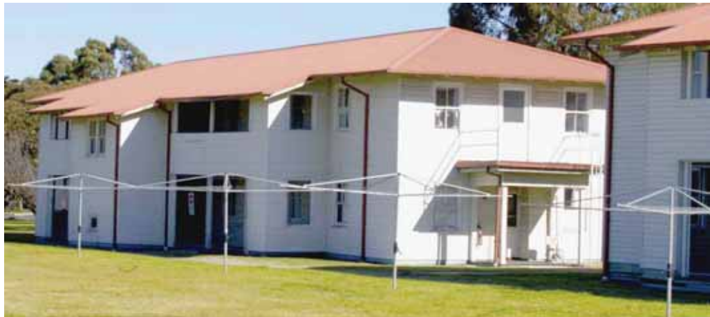
Photograph 3.22 Asset 41 – Mechanics' Quarters (Photograph courtesy DS-VT)
