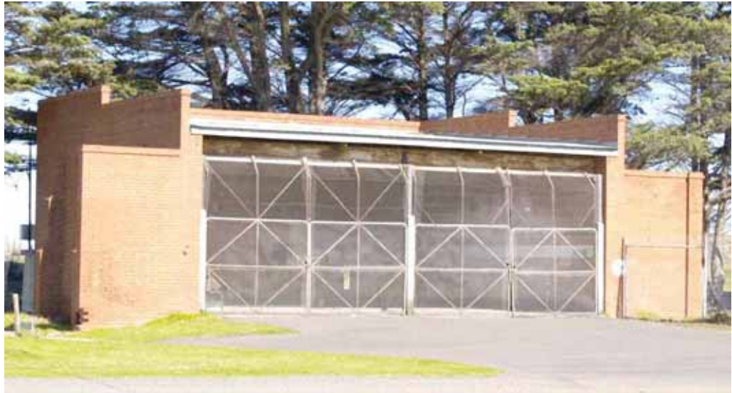
Photograph 3.11 Asset 224 – Stop Butt (Photograph courtesy DS-VT)
