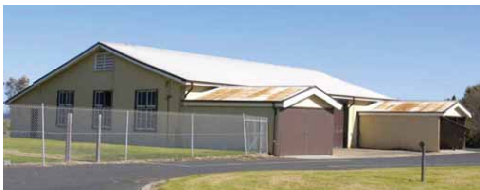
Photograph 3.1 Asset 90 – Warehouse (Photograph courtesy DS-VT)
