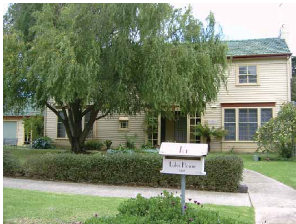
Photograph 3.16 Asset M027/28 - Lukis House (Photography by ERM 2007)
