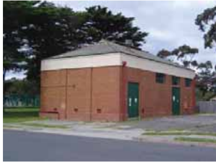
Photograph E.0.7 Substation No. 2 (Woodhead International, 2004)
