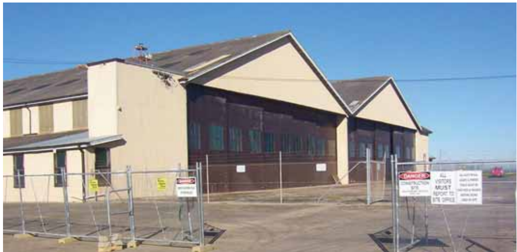
Photograph 3.4 Asset 101 – Seaplane Hangar (Photograph courtesy DS-VT)
