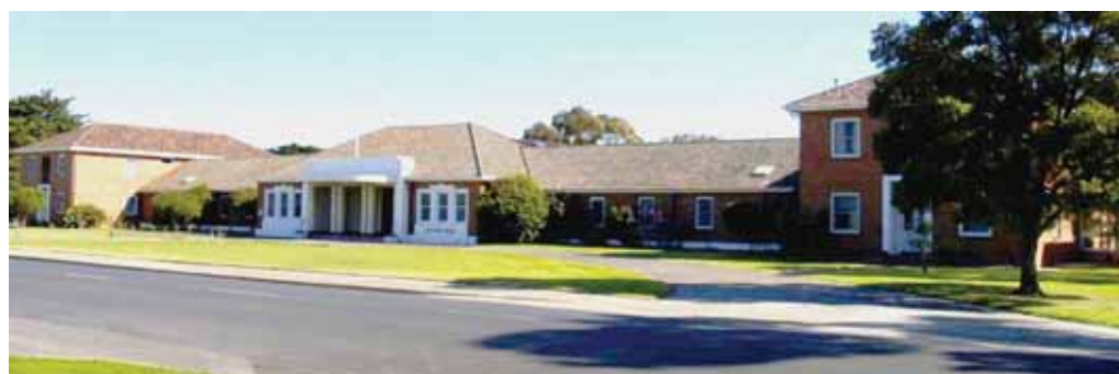
Photograph 3.26 Asset 33 – Officers' Mess (Photograph courtesy DS-VT)
