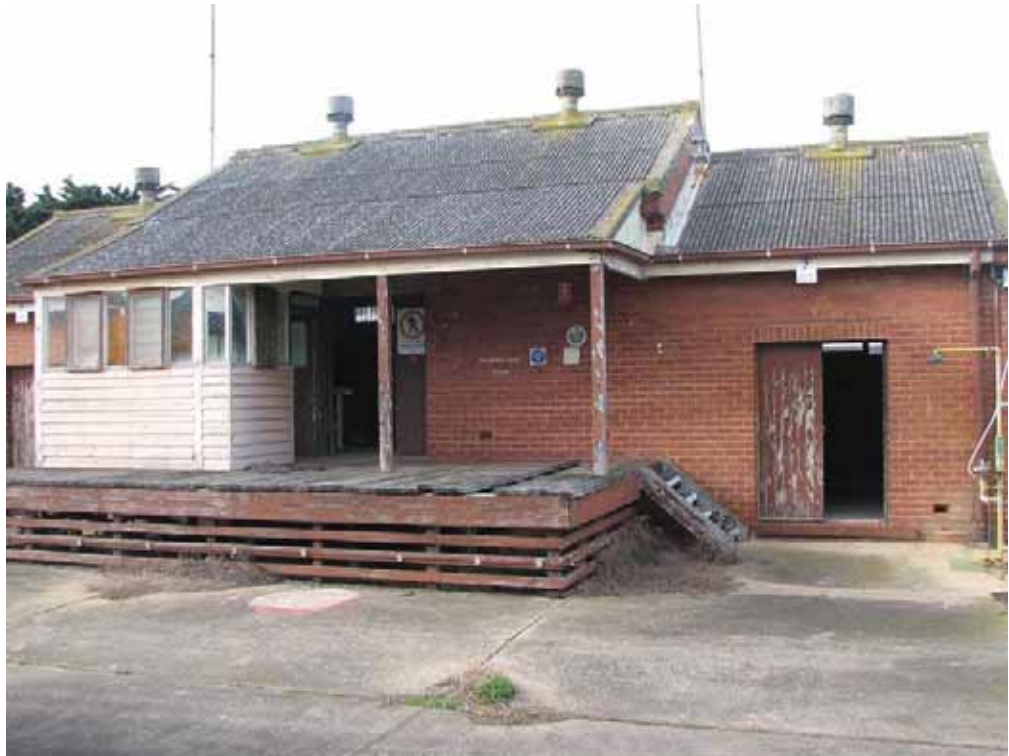
Photograph 3.8 Asset 122 - Hazardous / Inflammable Store (Photograph courtesy DS-VT)
