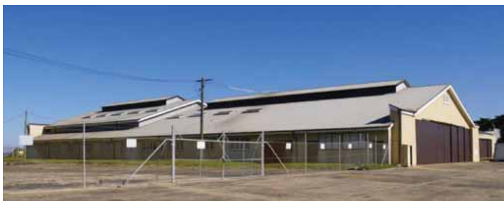
Photograph 3.2 Asset 95 – Hangar (Photograph courtesy DS-VT)
