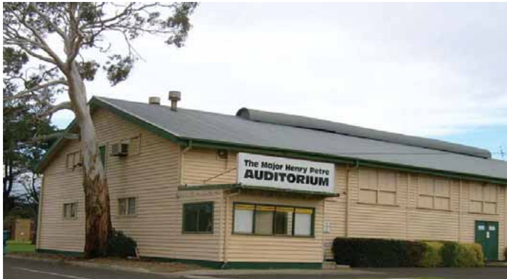
Photograph 3.21 Asset 38 – Major Henry Petre Auditorium (Photography by ERM 2007)
