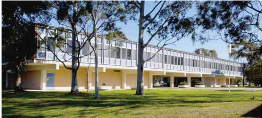
Photograph 3.24 Asset 10 – RAAF College (Photograph courtesy DS-VT)
