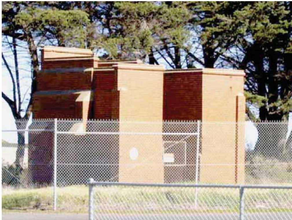
Photograph 3.7 Asset 121 - Gunnery Stop Butt (Photograph courtesy DS-VT)
