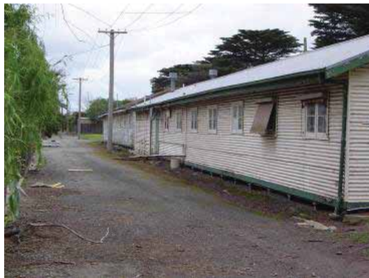
Photograph E.0.13 Buildings 158 and 156 – Note metal roof to 158 (Woodhead International, 2004)
