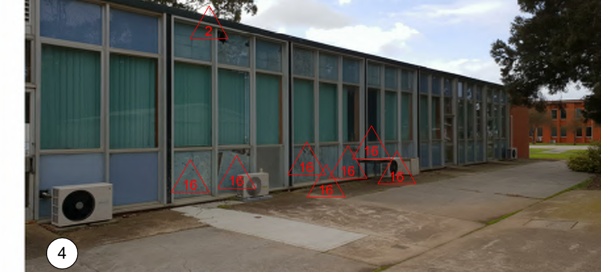
EXTERNAL SOUTH VIEW OF BUILDING
