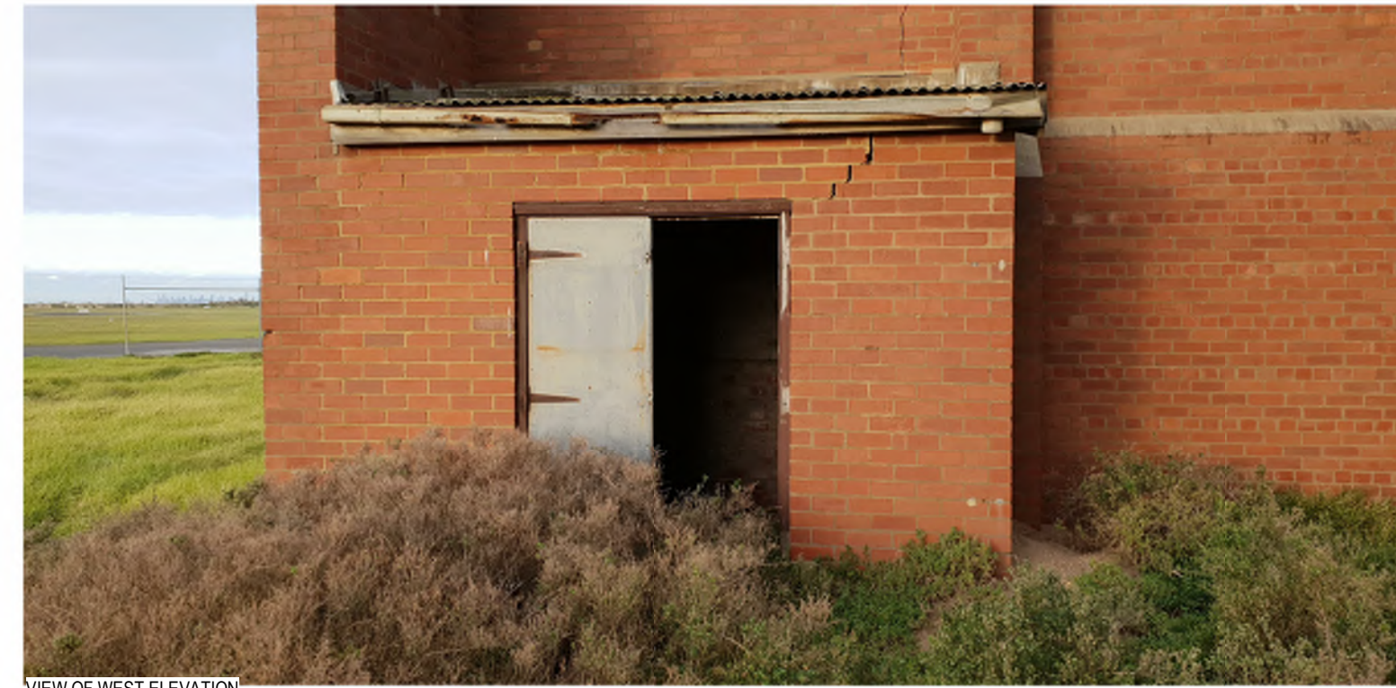
VIEW OF WEST ELEVATION
