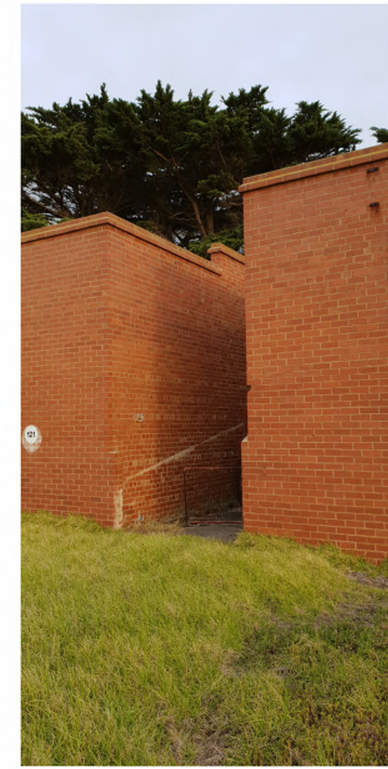
VIEW OUTSIDE THE STRUCTURE
