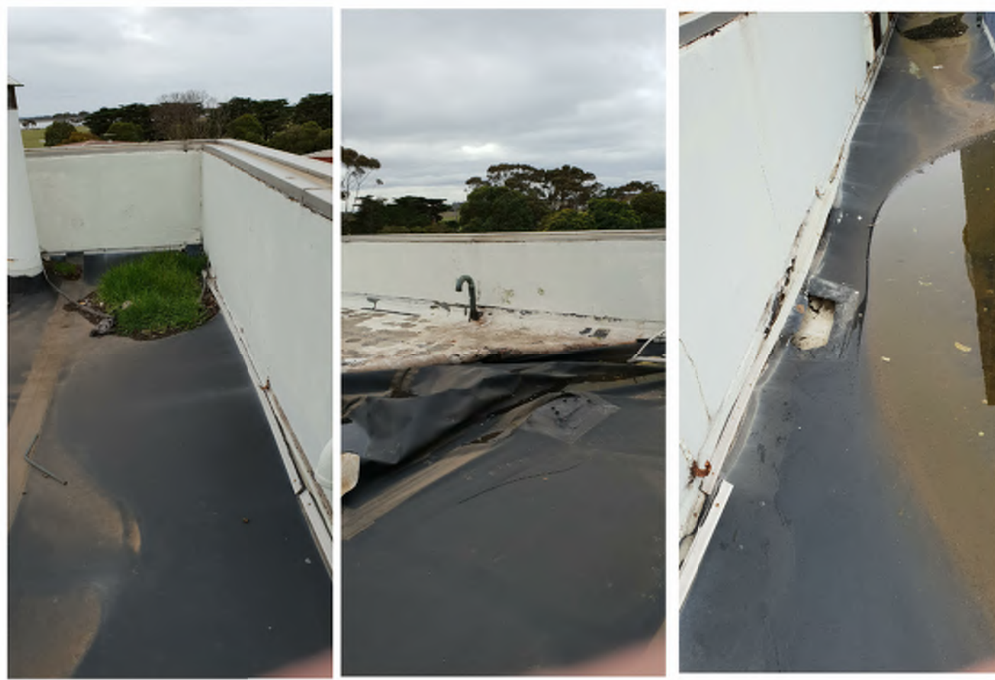
IMAGES OF DAMAGE TO WATERPROOF ROOF MEMBRANE
