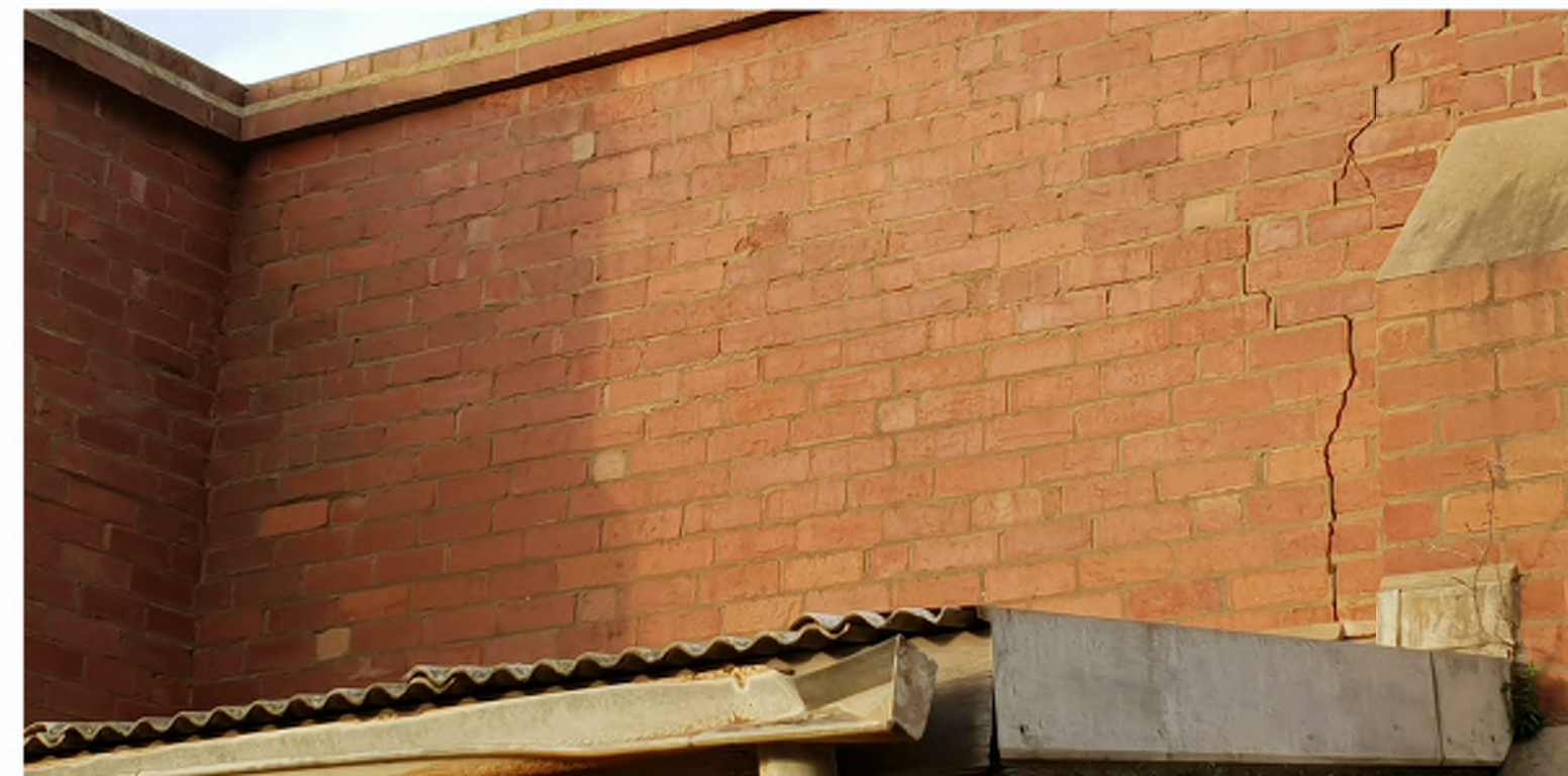
VIEW OF SHED ROOF
