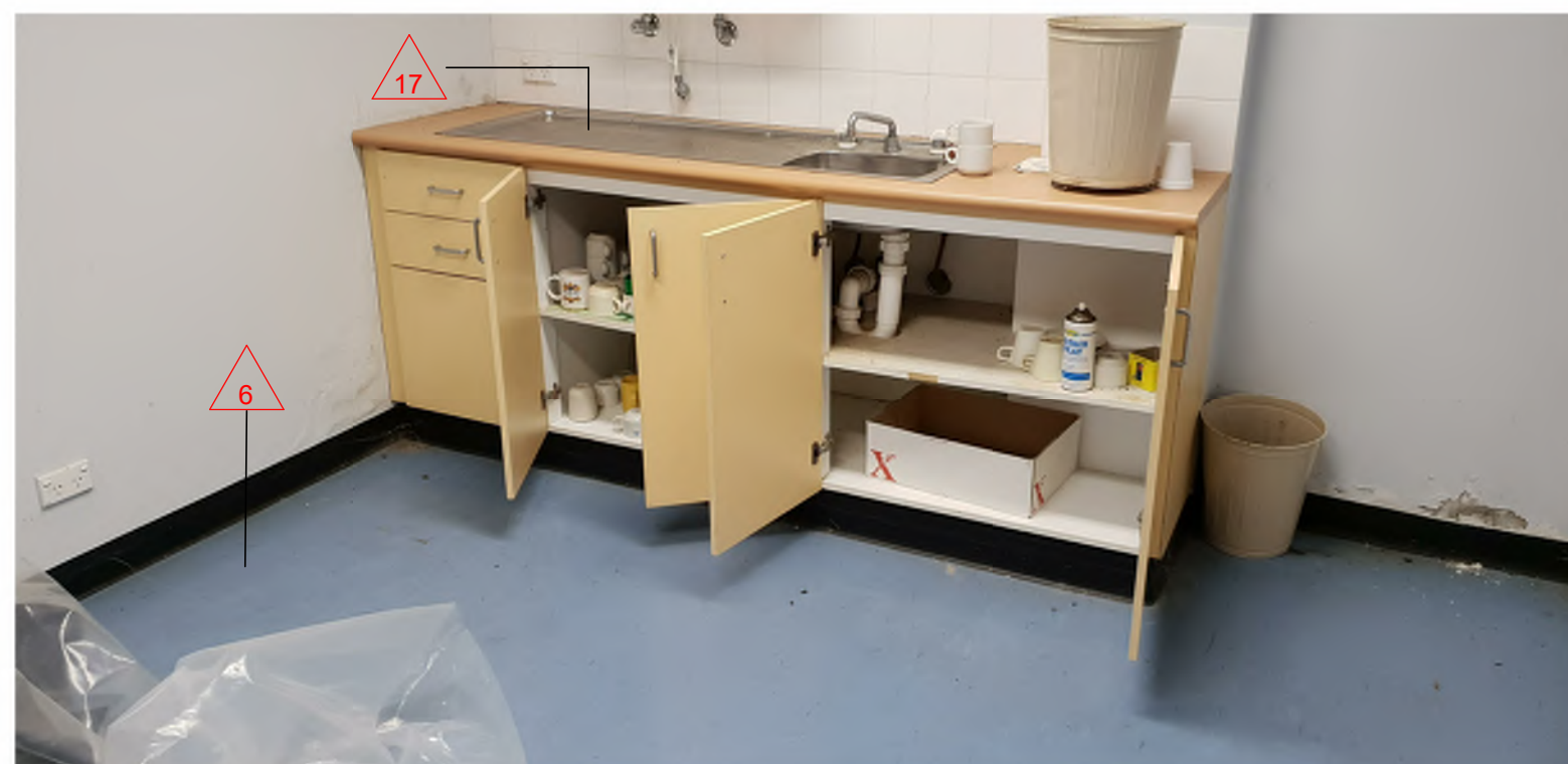
KITCHENETTE CARCASS SHOWING SIGNS OF WATER DAMAGE
