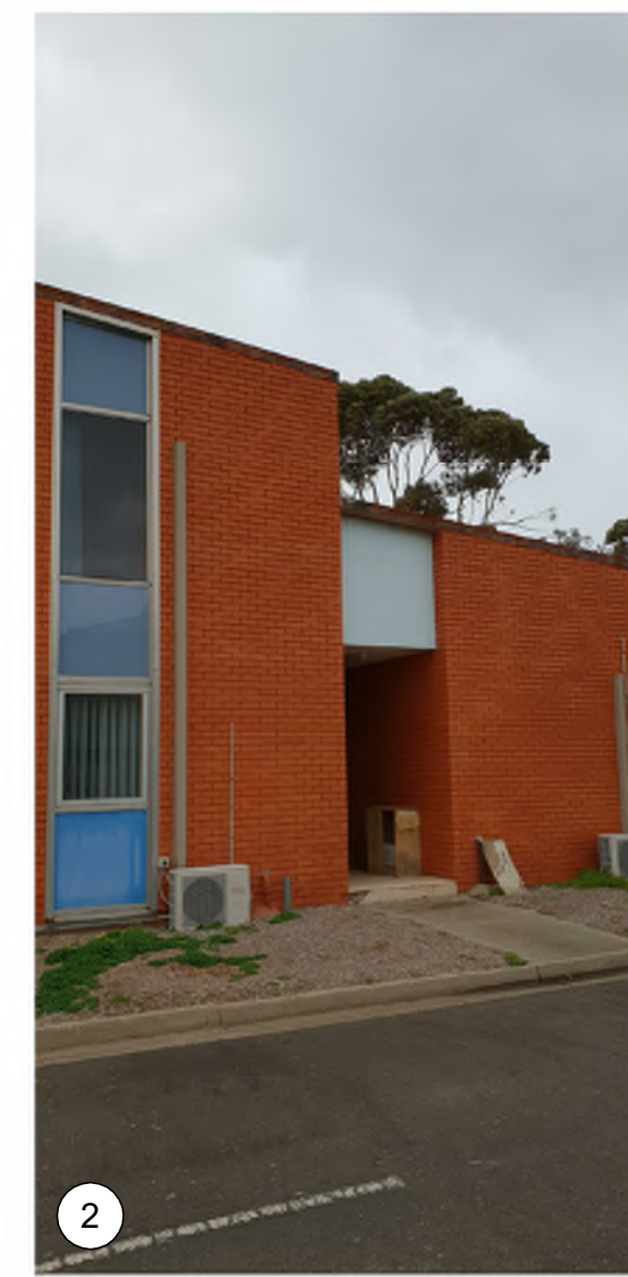
EXTERNAL VIEW OF BUILDING
