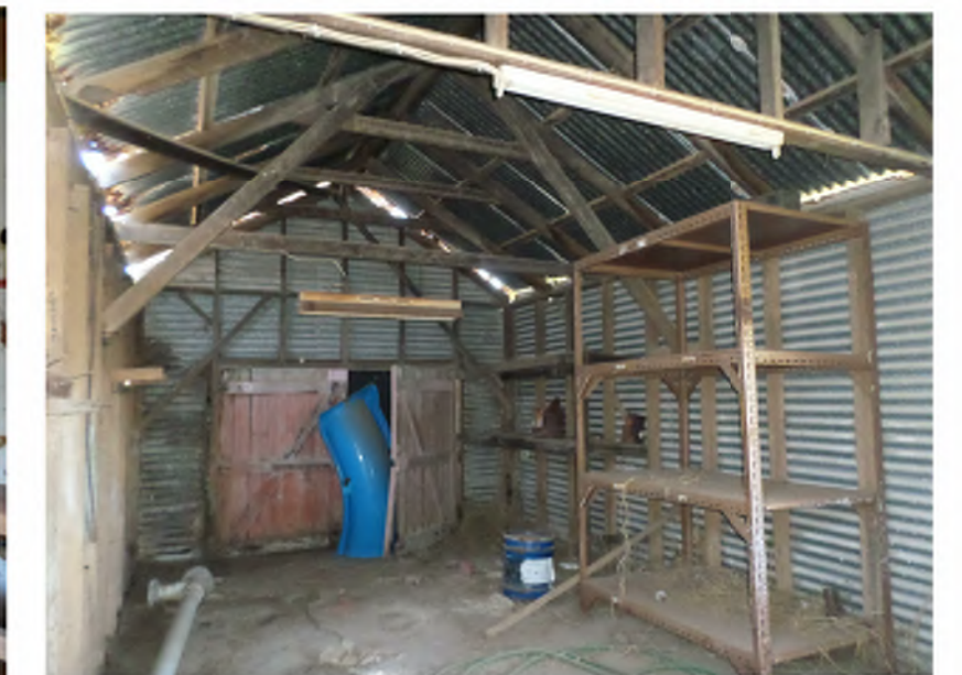
INTERNAL VIEW OF BUILDING 132
