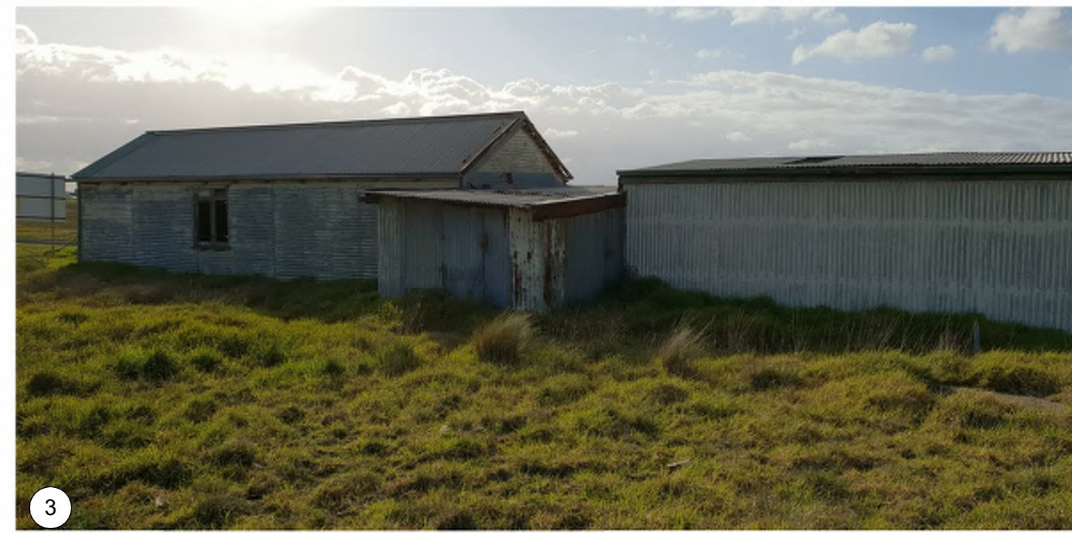
VIEW OF NORTH ELEVATION
