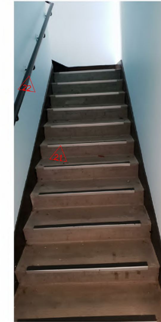
VIEW INTERNAL CONCRETE STAIRS
