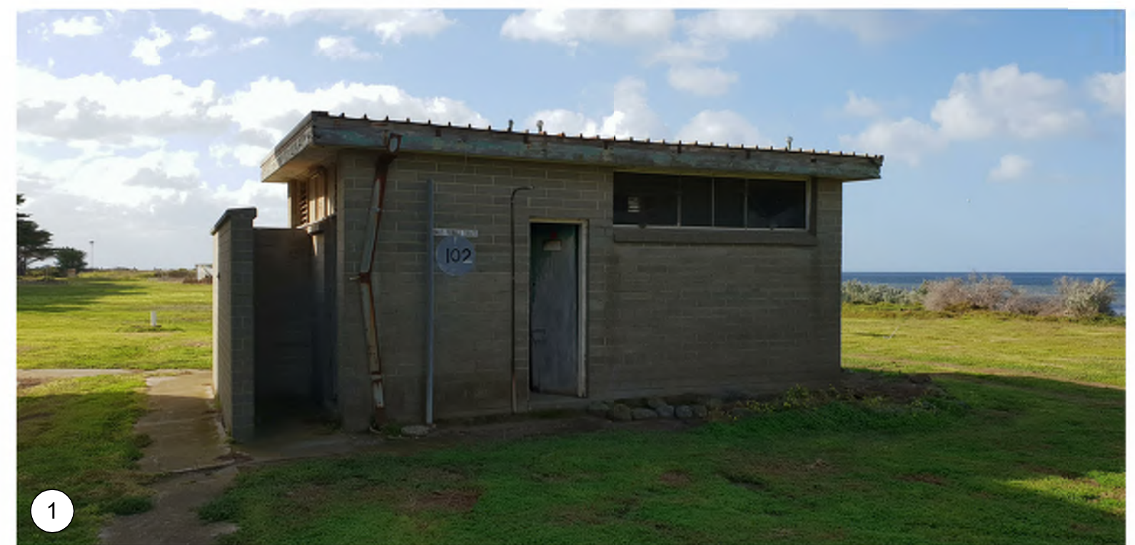
1 VIEW OF NORTH ELEVATION
