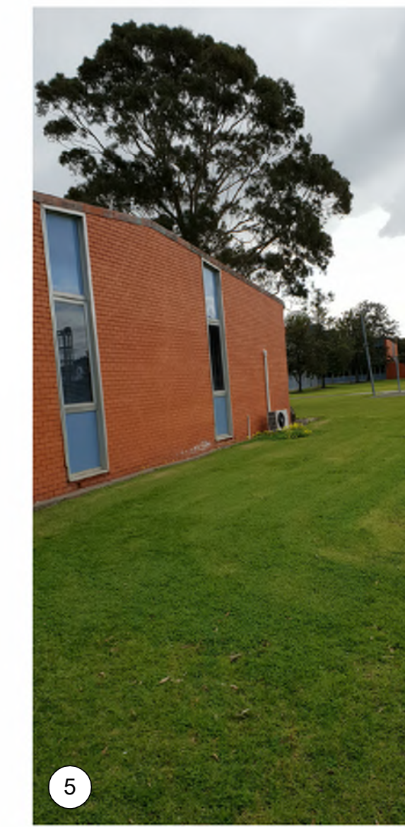
EXTERNAL VIEW OF BUILDING
