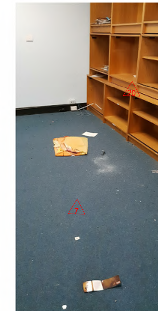
TYPICAL VIEW OF UPPER LEVEL
