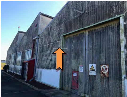
Photo 1. Asbestos-containing corrugated cement to walls.
