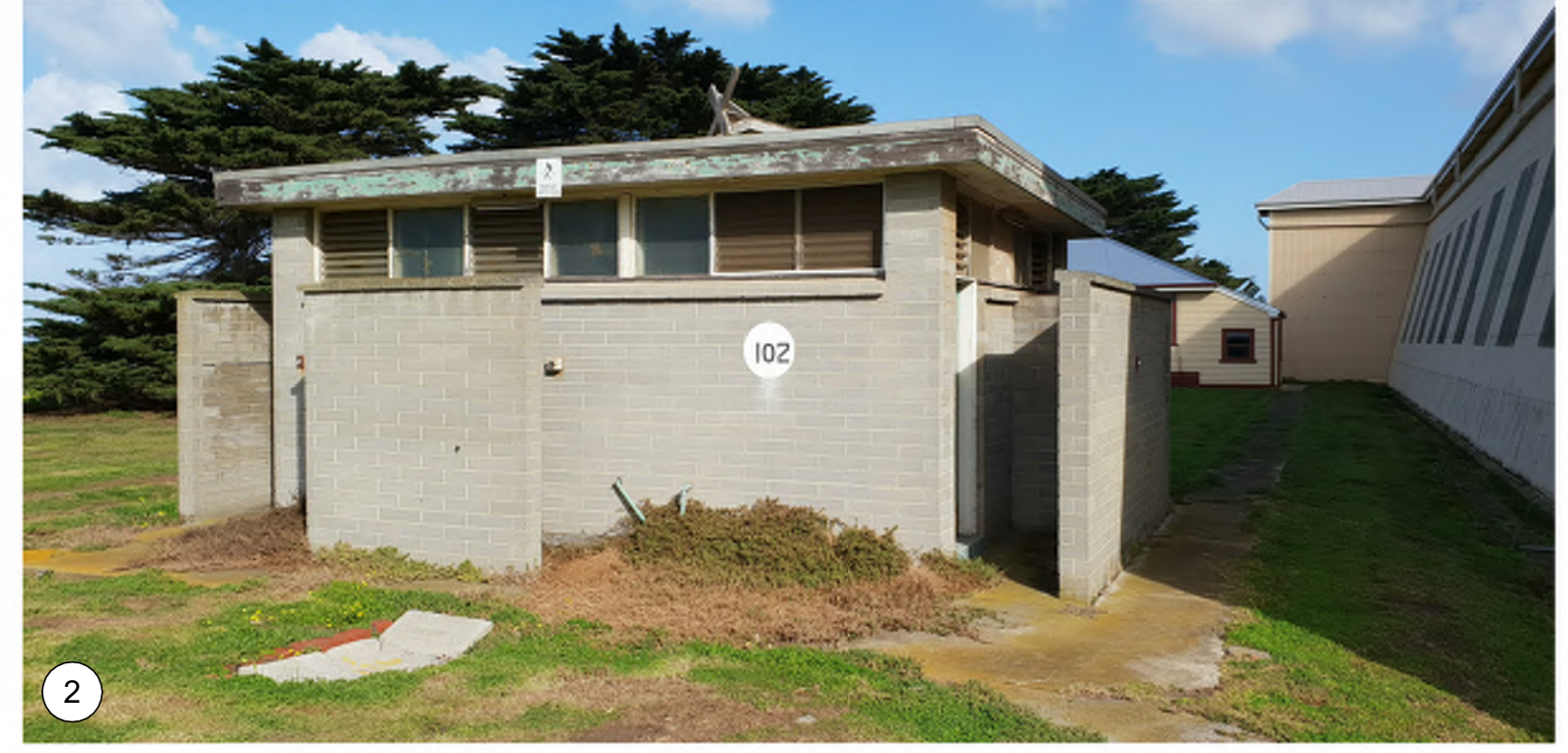
2 VIEW OF EAST ELEVATION
