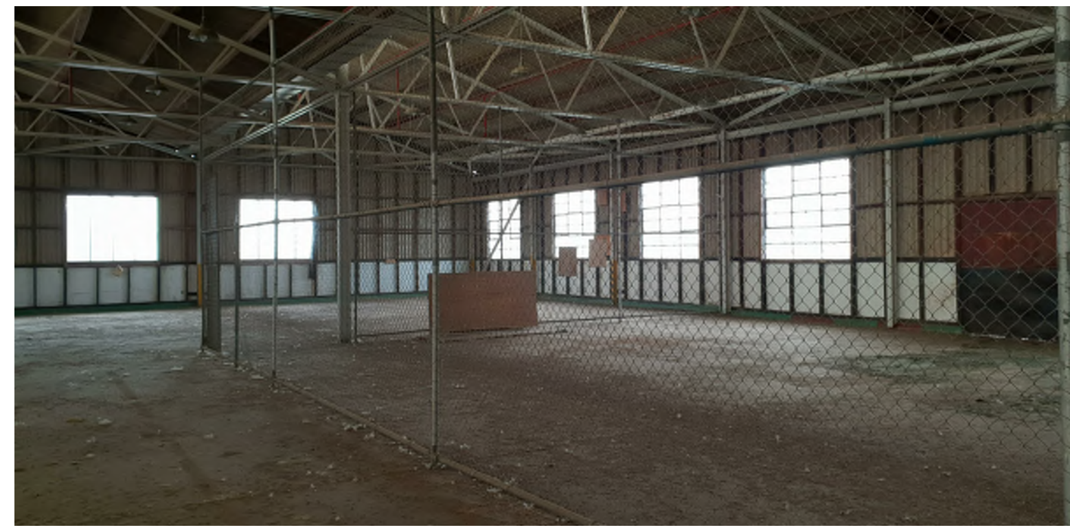
INTERNAL CAGED STORE AREA TO BE DEMOLISHED
