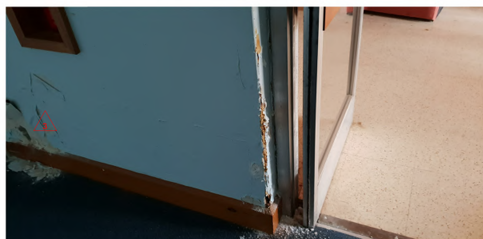
TYPICAL INTERNAL WALL TO BE REPAIRED, PATCHED AND PAINTED
