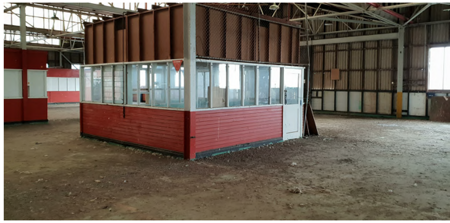
TYPICAL INTERNAL OFFICE TO BE DEMOLISHED
