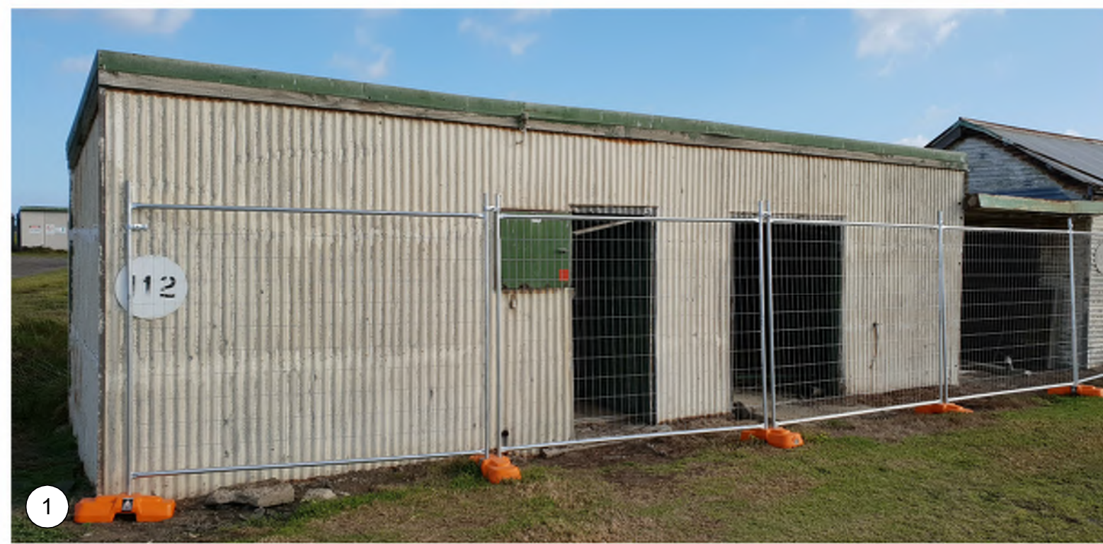
VIEW OF SOUTH ELEVATION - BUILDING 112
