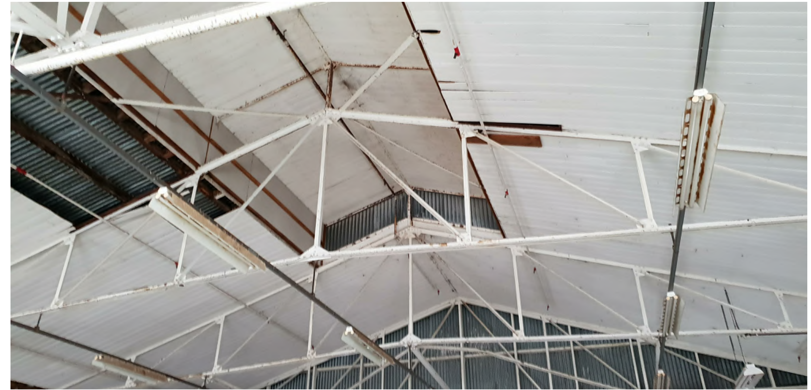
TYPICAL IMAGES - INTERNAL STEEL STRUCTURE / DUTCH GABLE
