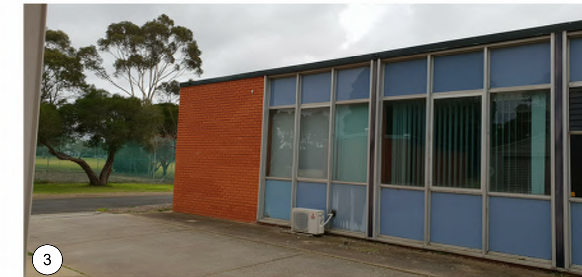
EXTERNAL SOUTH VIEW OF BUILDING
