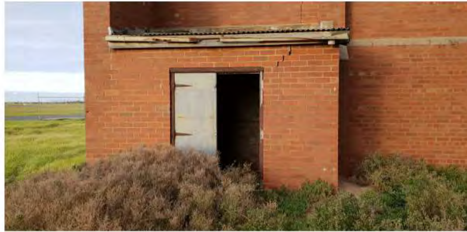
PHOTO NO 2 - VIEW OF WEST ELEVATION
