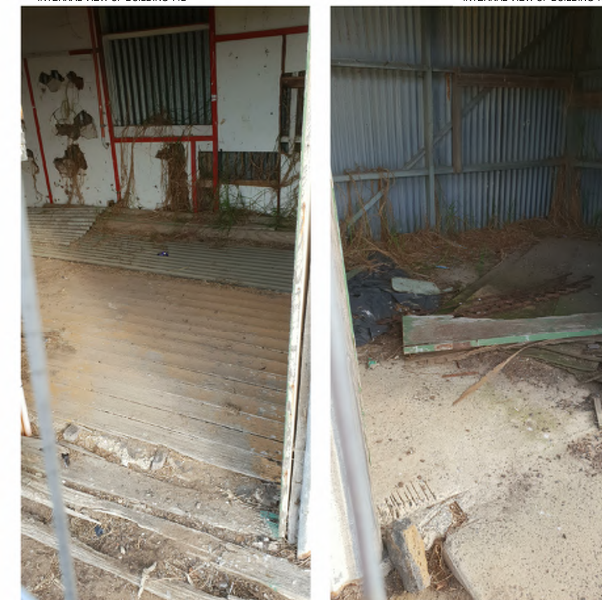
INTERNAL VIEW OF BUILDING 112
