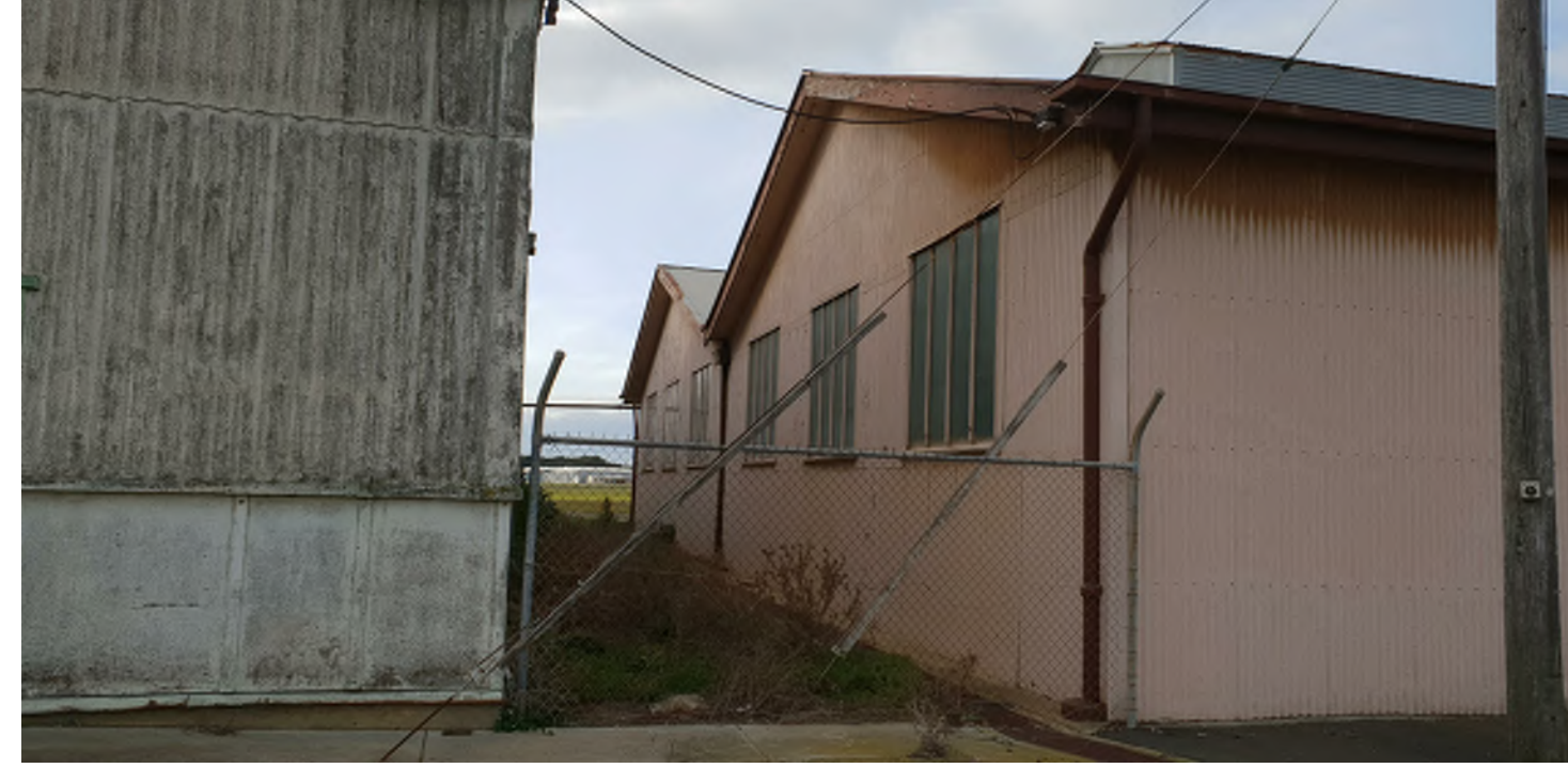
TYPICAL IMAGES - EXTERNAL/ ADJOINING BUILDING
