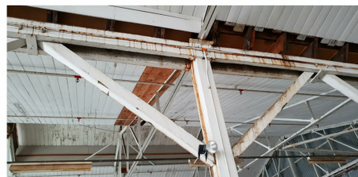
TYPICAL IMAGES - CEILING LININGS
