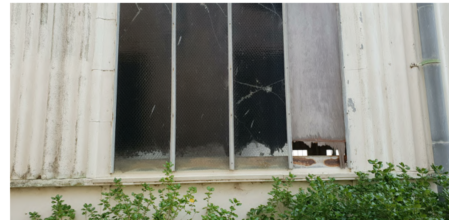
EXISTING STEEL FRAMED WINDOWS TO BE REPLACED
