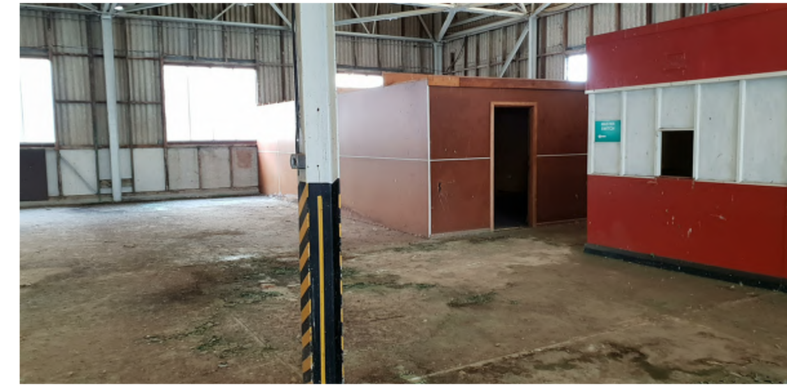
INTERNAL OFFICES TO BE DEMOLISHED
