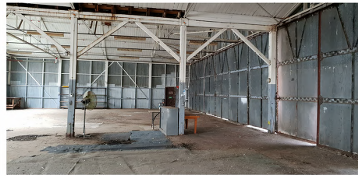
TYPICAL IMAGES - CONCRETE SLAB/ BUILDING STRUCTURE
