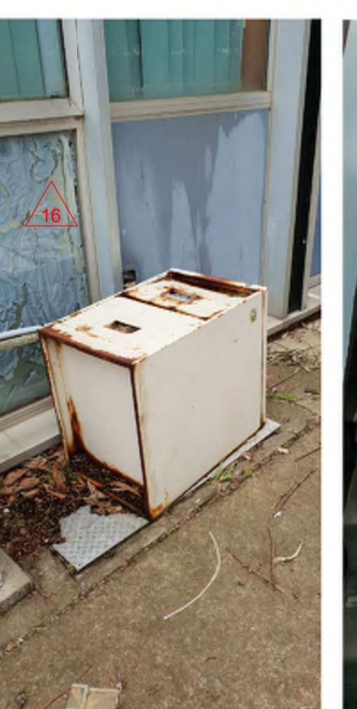
SCOPE 16 - CRACKED GLAZING TO BE REPLACED
