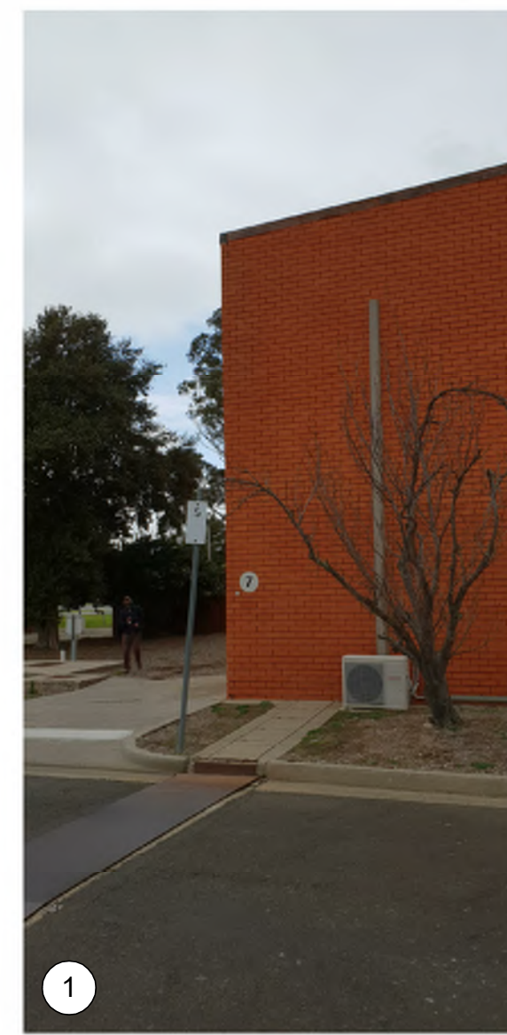
EXTERNAL VIEW OF BUILDING
