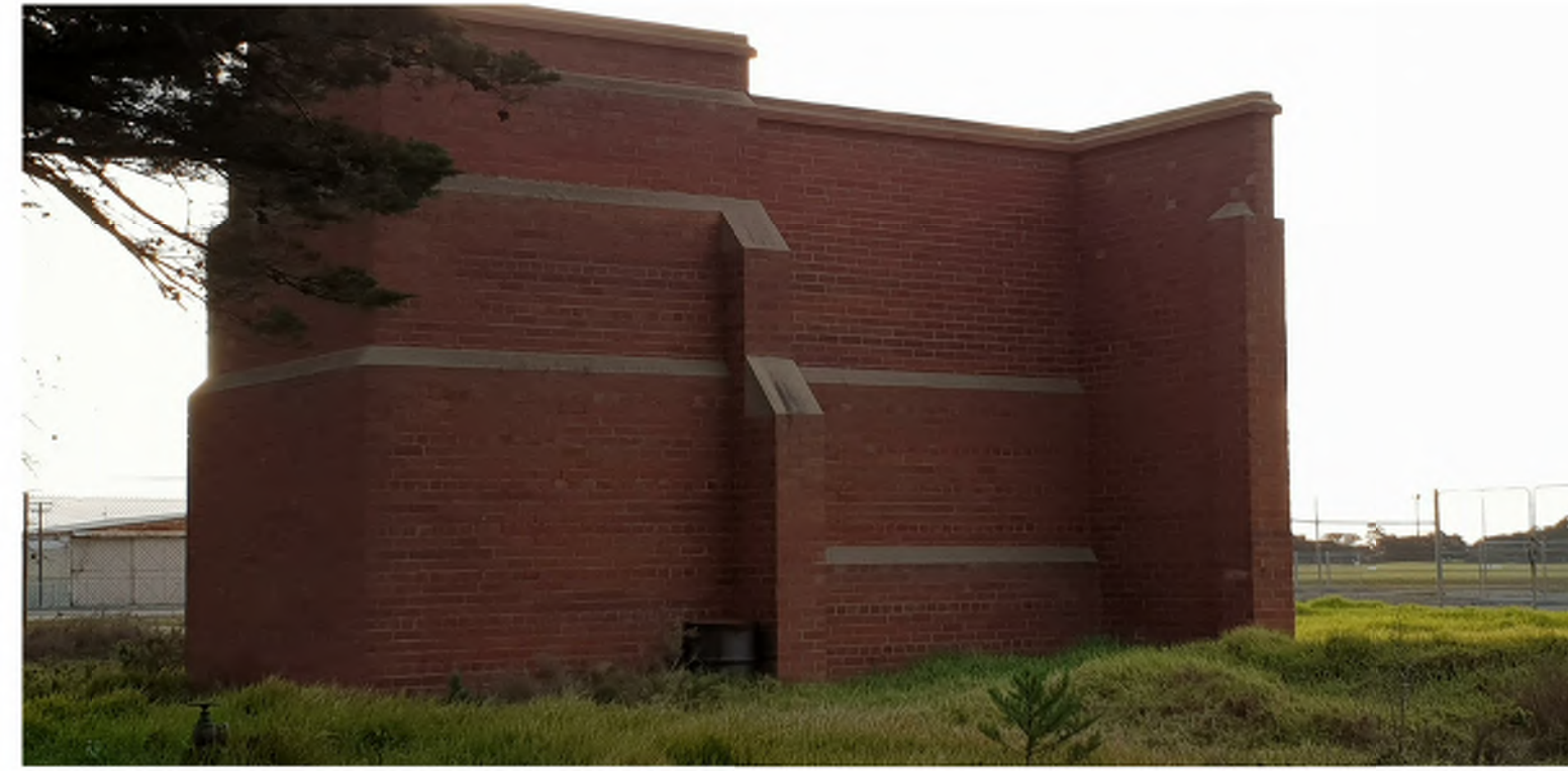
VIEW OF EAST ELEVATION
