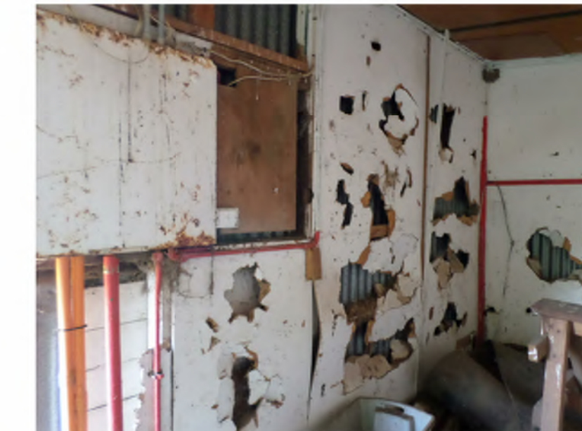
INTERNAL VIEW OF BUILDING 112
