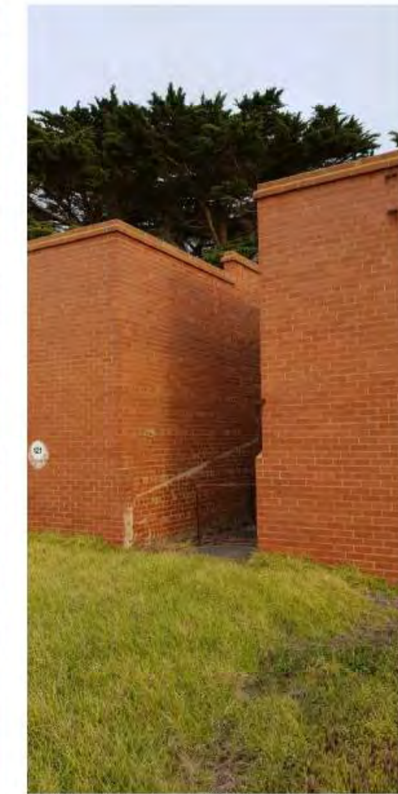
PHOTO NO 6 - VIEW OUTSIDE THE STRUCTURE, WITH VEGETATION TO BE REMOVED
