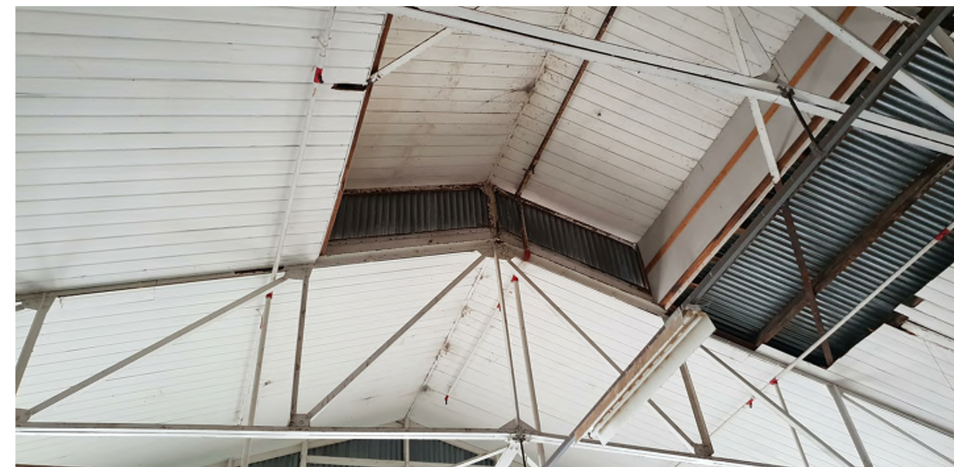
TYPICAL IMAGES - CEILING LININGS
