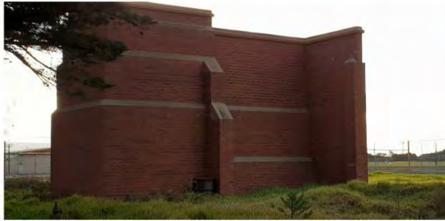
PHOTO NO 1 - VIEW OF EAST ELEVATION
