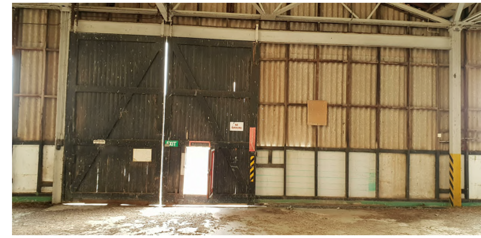
EXISTING LARGE TIMBER DOORS TO BE REPLACED
