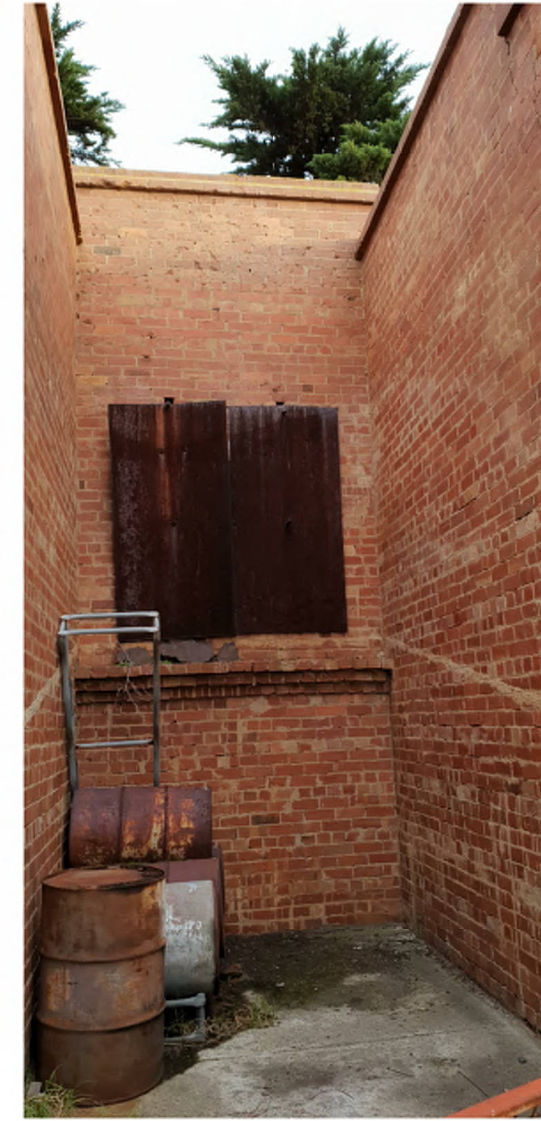
VIEW INTO THE STRUCTURE
