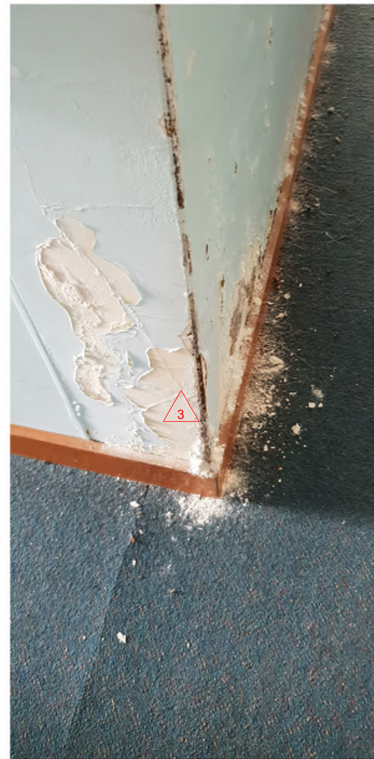
SCOPE 3 - IMAGE OF TYPICAL INTERNAL WALLS DAMAGE TO BE PATCHED AND PAINTED
