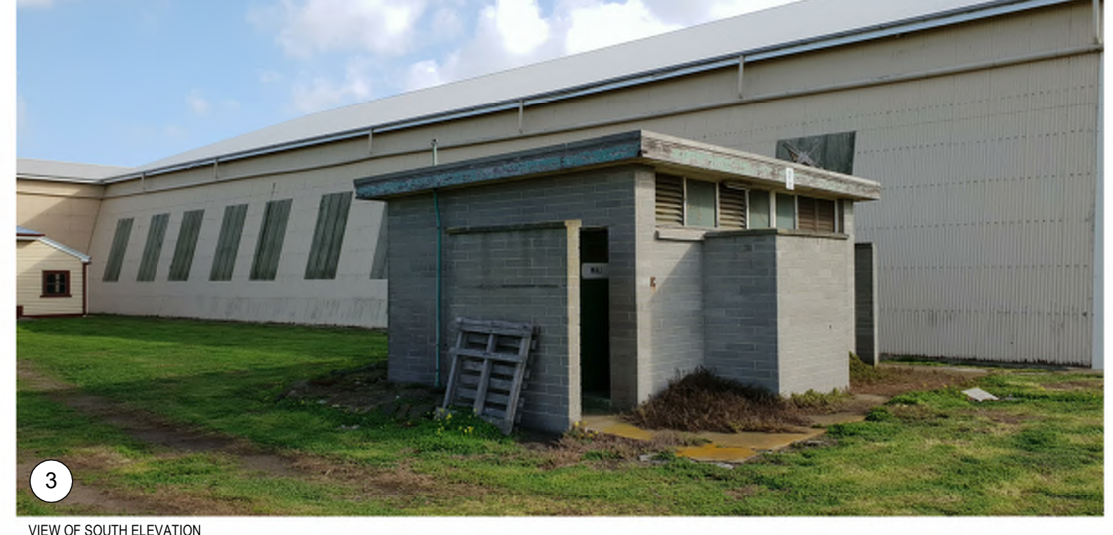
3 VIEW OF SOUTH ELEVATION
