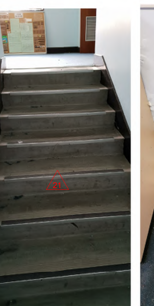
SCOPE 21 - CONCRETE STAIRS TO BE CLEANED, SEALED AND TACTILE INDICATORS APPLIED
