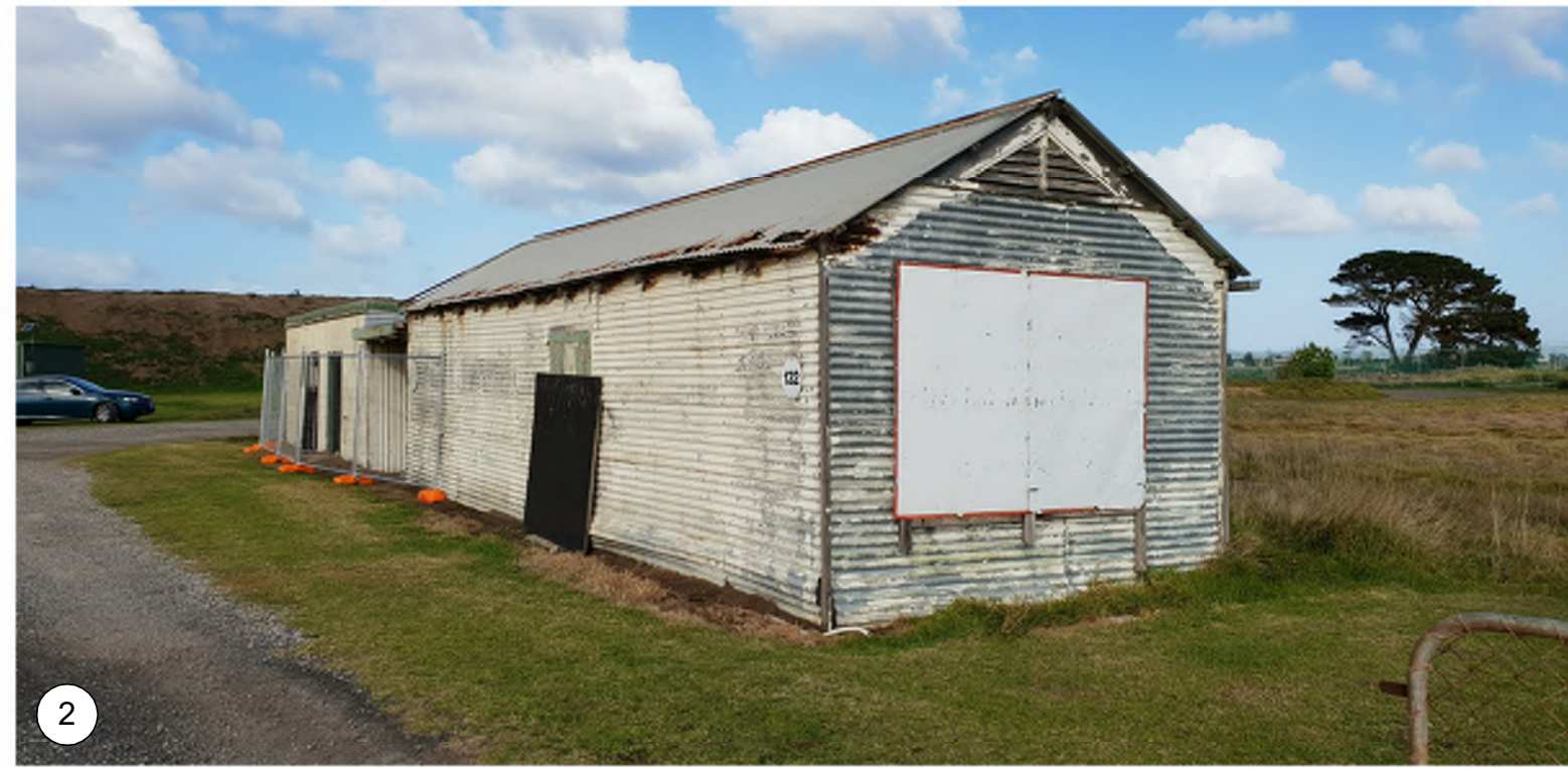
VIEW OF EAST ELEVATION - BUILDING 132
