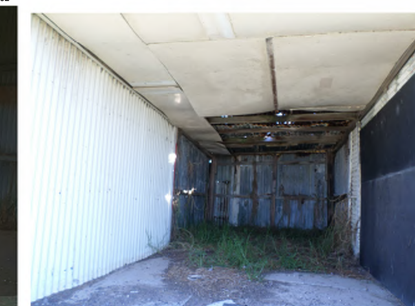
INTERNAL VIEW OF UNDERCOVER AREA BETWEEN BUILDING 112/ 132
