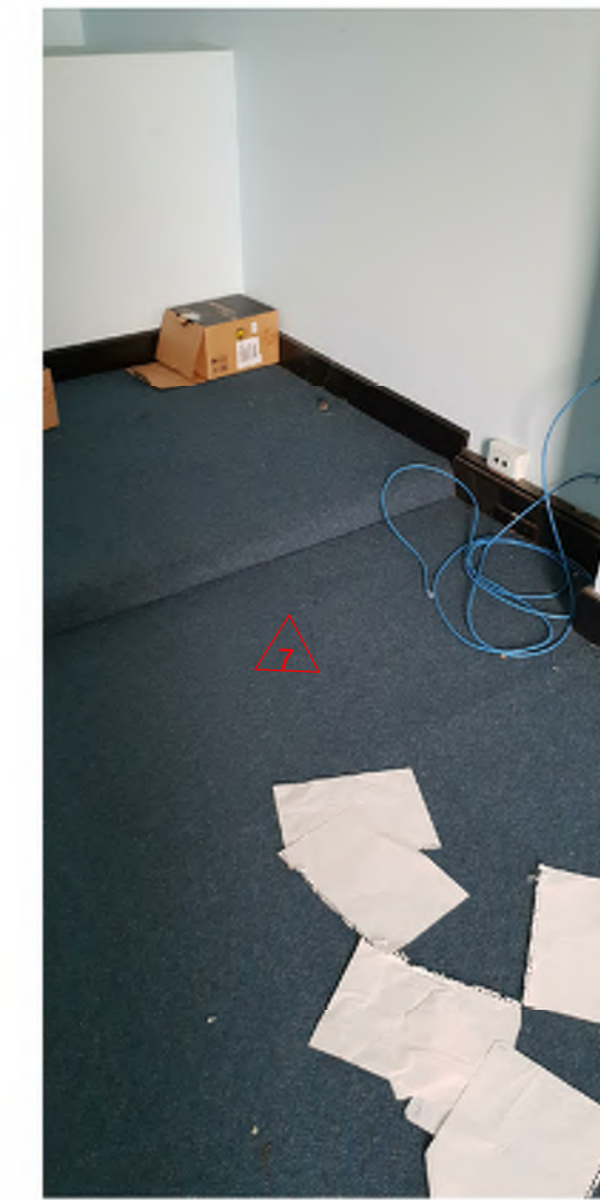
TYPICAL VIEW OF UPPER LEVEL
