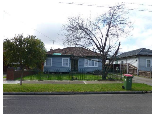
Figure 12 68 Wellington Street, West Footscray
