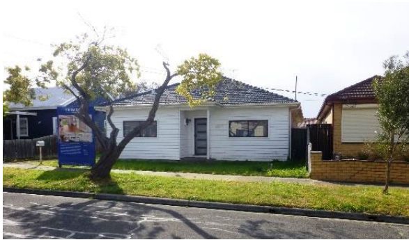
Figure 13 76 Wellington Street, West Footscray
