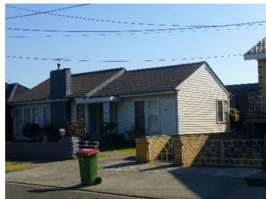
Figure 11 62 Wellington Street, West Footscray
