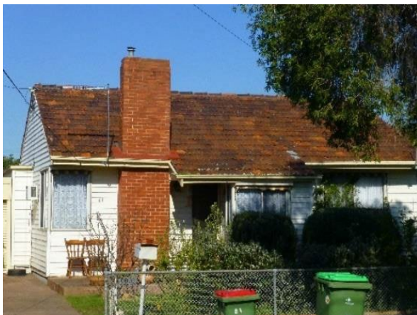
Figure 10 61 Wellington Street, West Footscray
