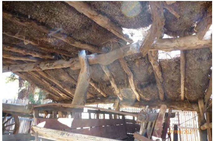
2021, Holes in thatched roof of Pole Stable
