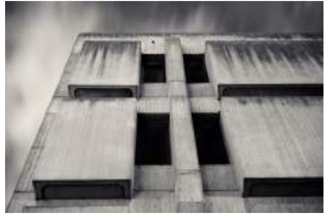
1.8 Footscray Psychiatric Centre concrete detail. Note the board-marked concrete and the underside lip of the precast projecting wall panels, and the deep inset of the windows. Photo: John Jovic.
