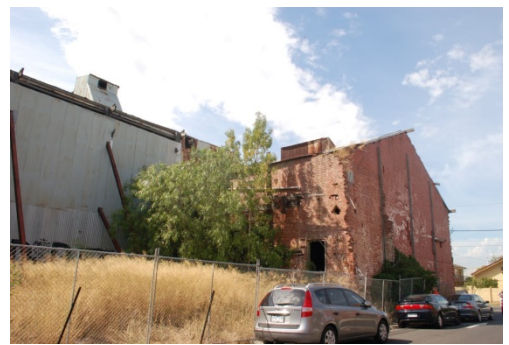
The west elevation of the brick pressing shed and former engine house
