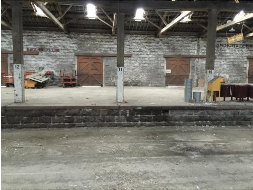
Figure 15 Interior of shed, showing loading platform and lowered central rail tracks
