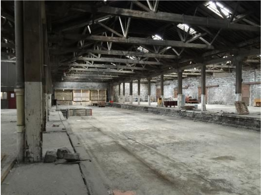
Figure 14 Interior of shed, looking east
