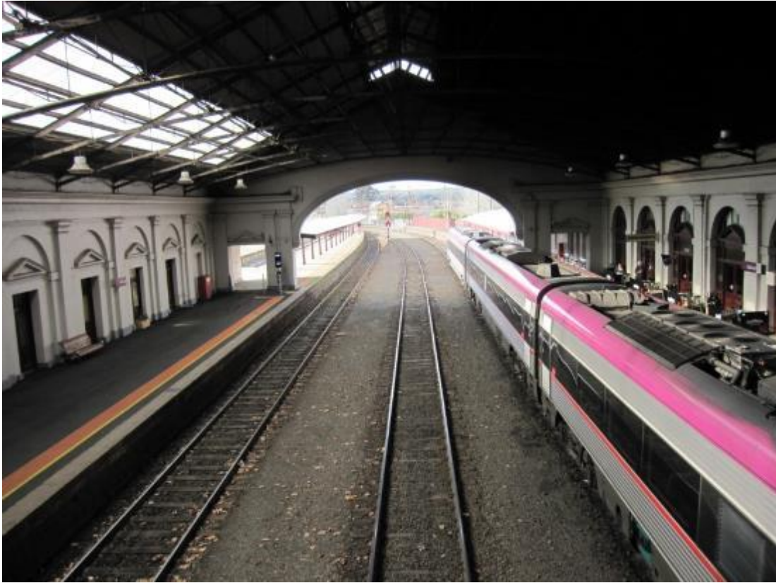
Figure 35 Train hall, with north station building at left, and south station building at right
