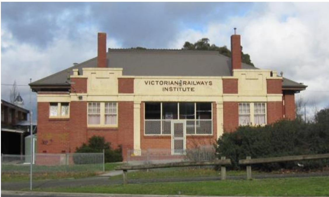
Figure 40 VRI building, north-west corner of railway reserve
