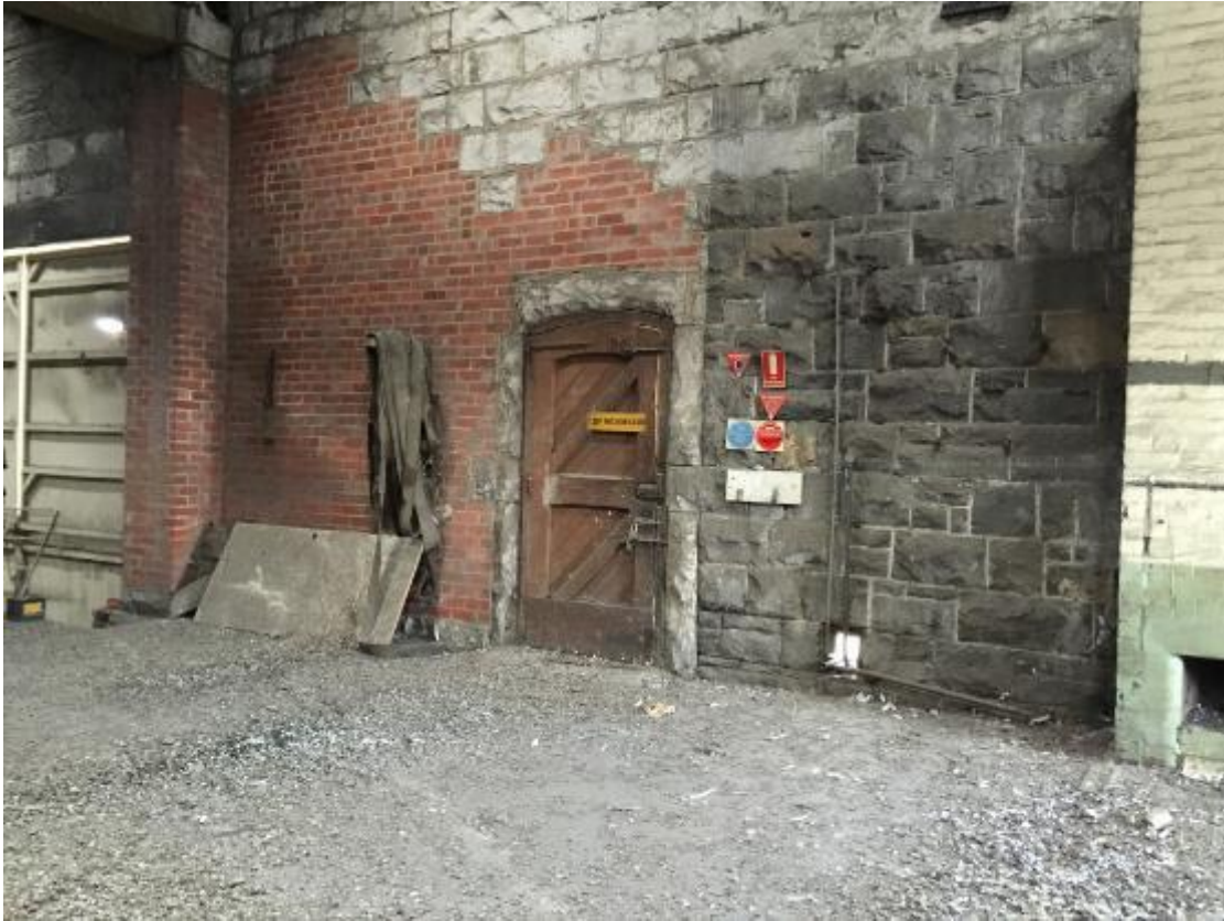
Figure 17 Internal wall showing later brick infill
