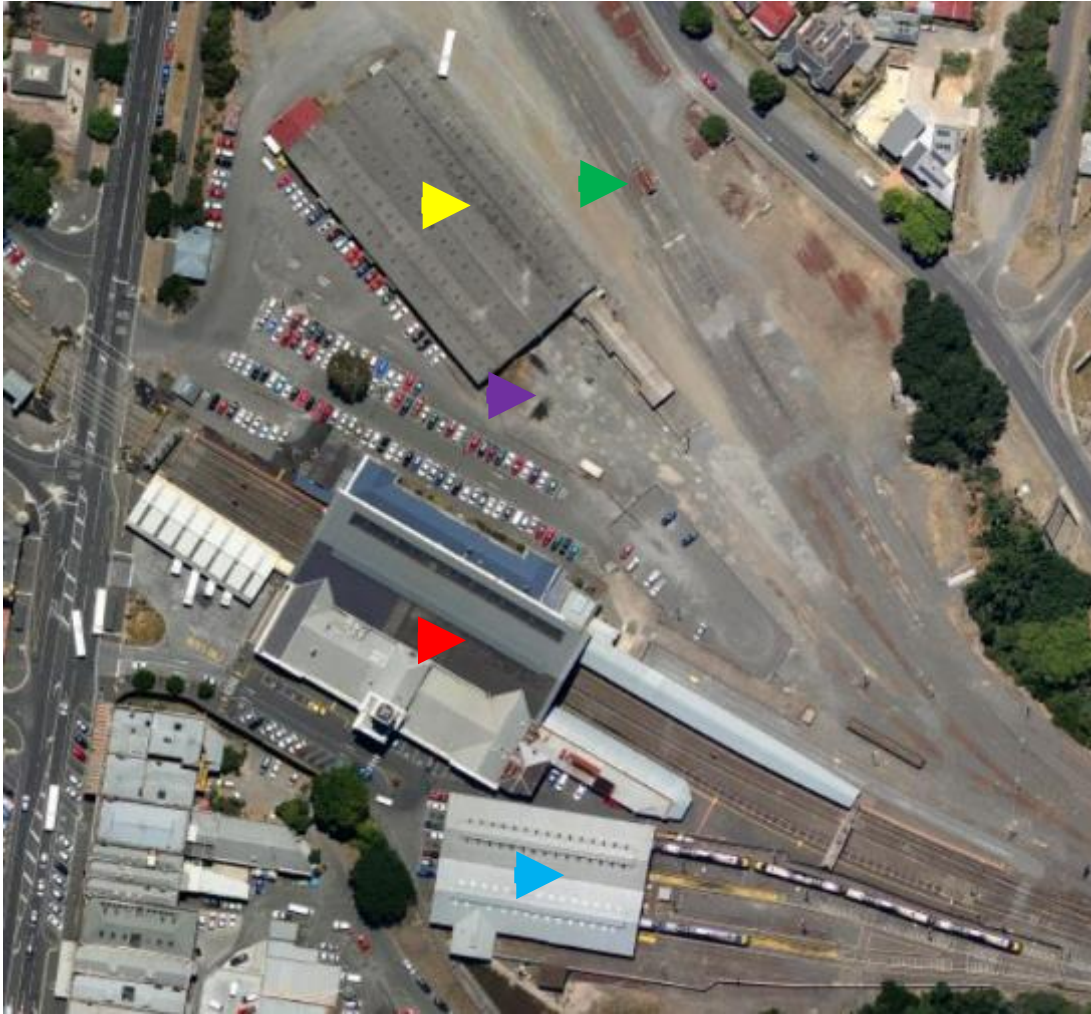
Figure 4 Aerial image of Ballarat Station, showing the Goods Shed (yellow arrow), combined north station building/train hall/south station building (red arrow), engine shed (blue arrow) and site of weighbridge showing small office building which has since been demolished (green arrow). The purple arrow indicates the approximate location of an underground space, abutting the south-east corner of the Goods Shed. Lydiard Street North is at left. Source: Nearmap
