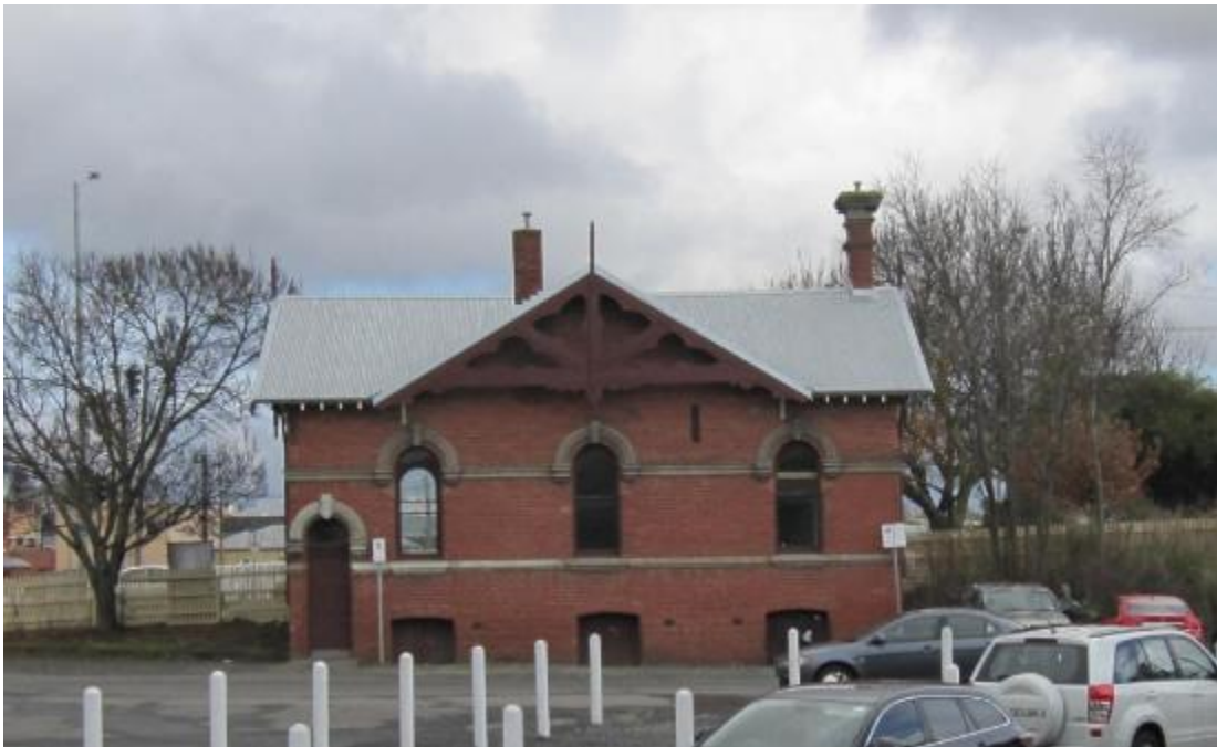
Figure 36 Carrier's office, east elevation
