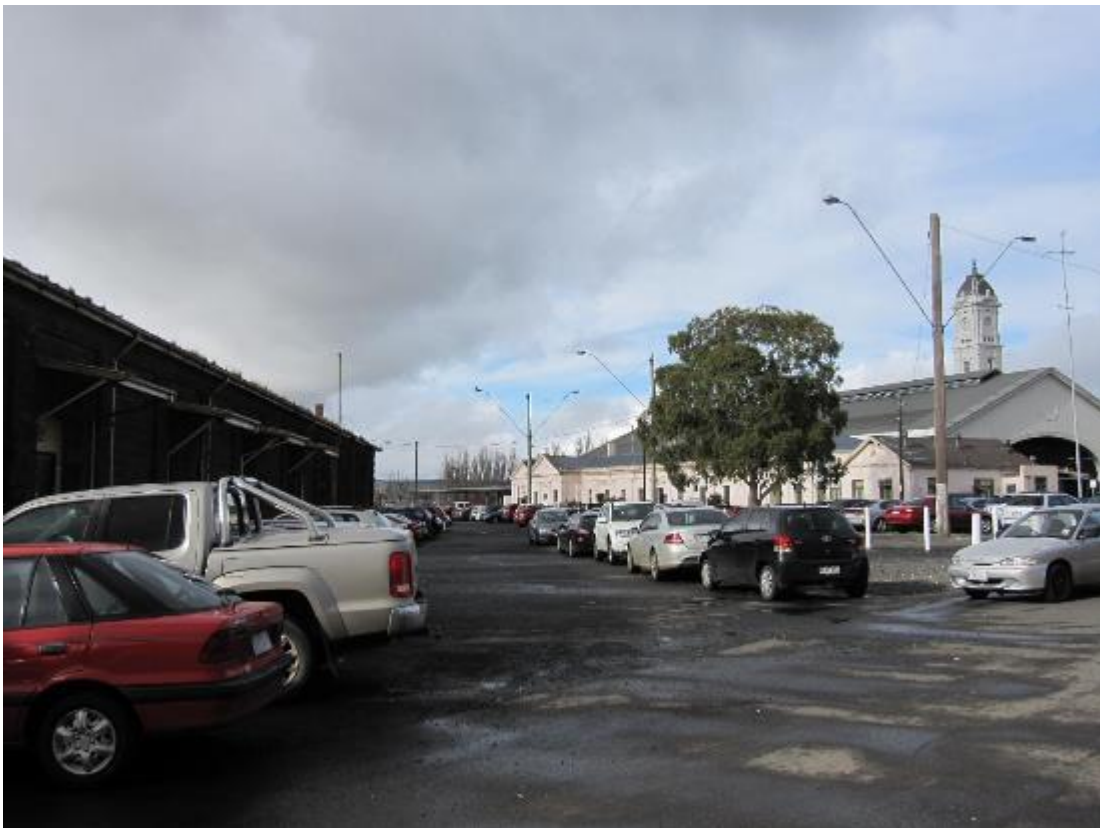
Figure 26 Landscape between Goods Shed and north station building, looking east
