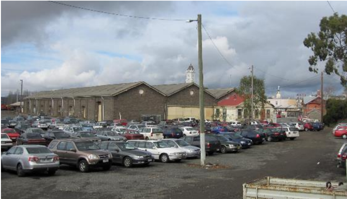
Figure 5 Goods Shed showing west gabled end and long north elevation (at left)
