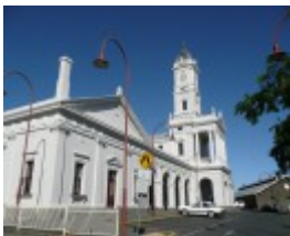
BALLARAT RAILWAY COMPLEX SOHE 2008
