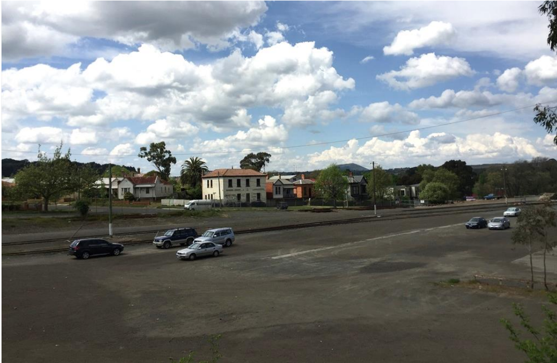
Figure 25 Northern area of railway reserve with Nolan Street in the distance; the Goods Shed is out of view at right; the hotel will be constructed in the left of image
