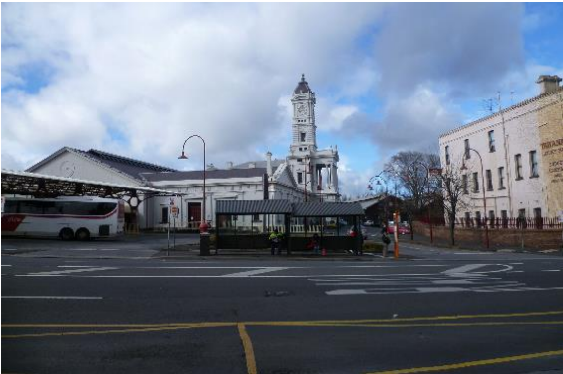
Figure 31 Ballarat Station as seen from Lydiard Street North
