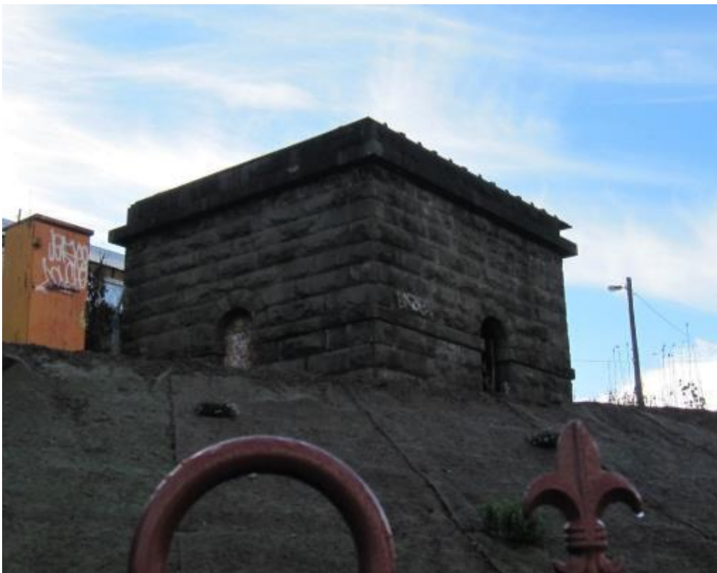
Figure 42 Water tank, south side of engine shed
