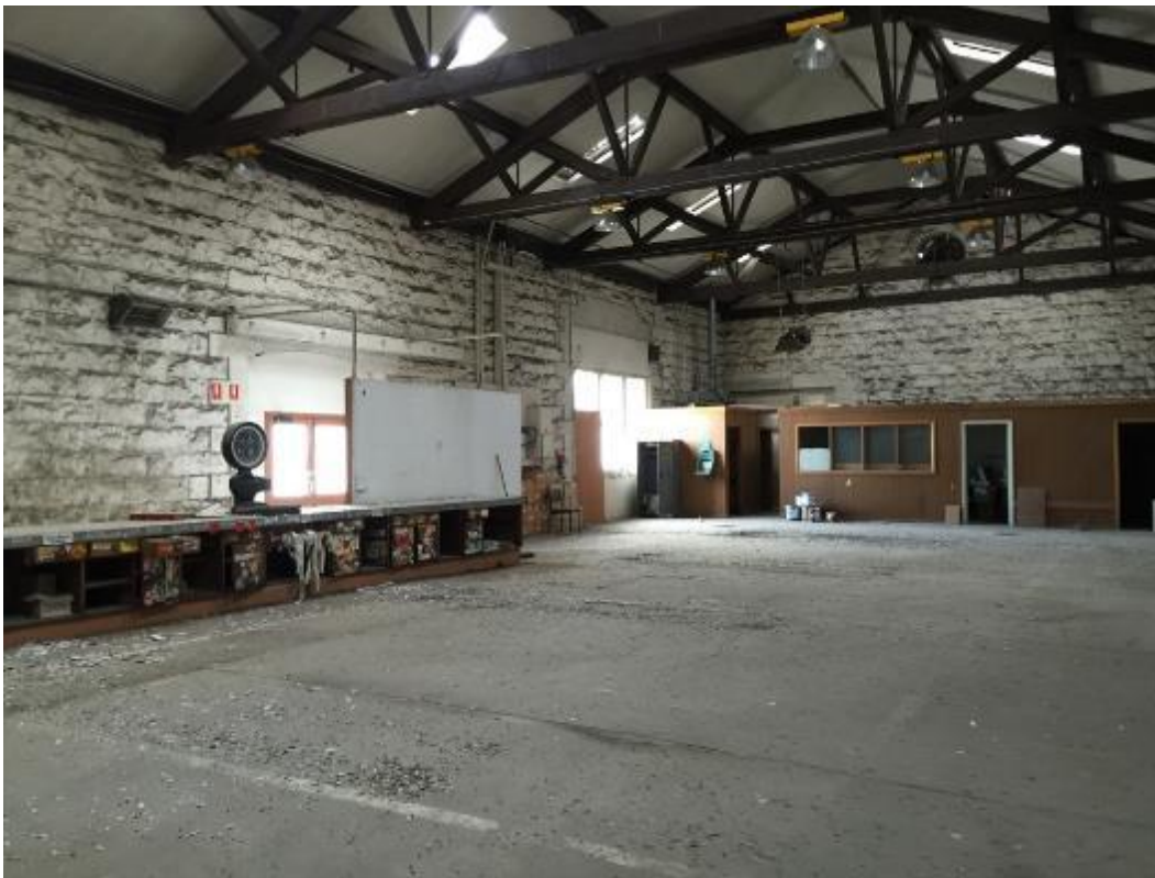
Figure 16 Interior of shed, looking west
