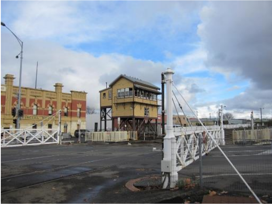
Figure 43 Boom gates, Lydiard Street North
