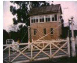
ballarat railway complex signal box & gates
