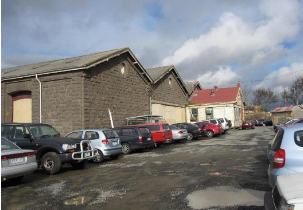
Figure 7 Another view of the west gabled end, with timber addition to the far (right) gable proposed for removal
