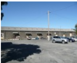
BALLARAT RAILWAY COMPLEX SOHE 2008
