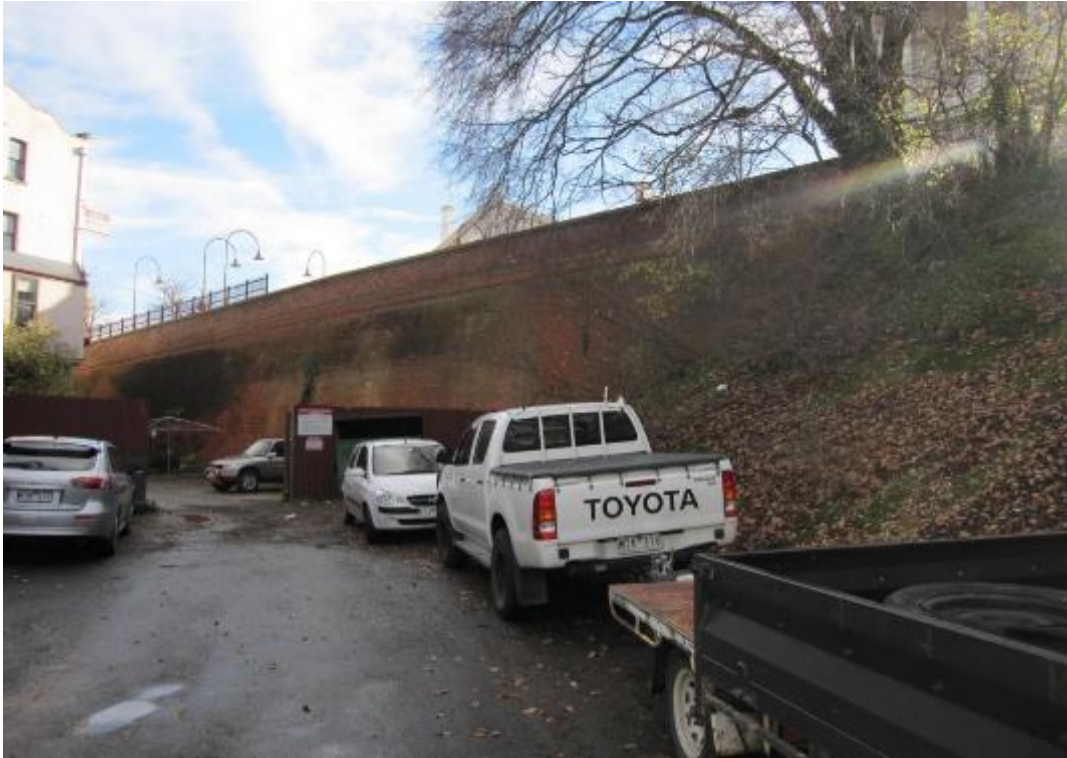
Figure 45 South side of railway reserve, showing embankment and retaining wall
