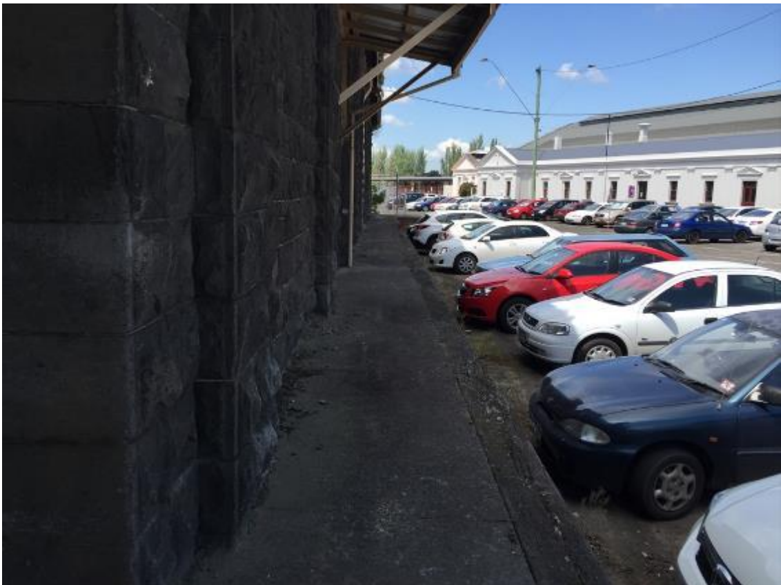
Figure 12 Detail of platform to south elevation
