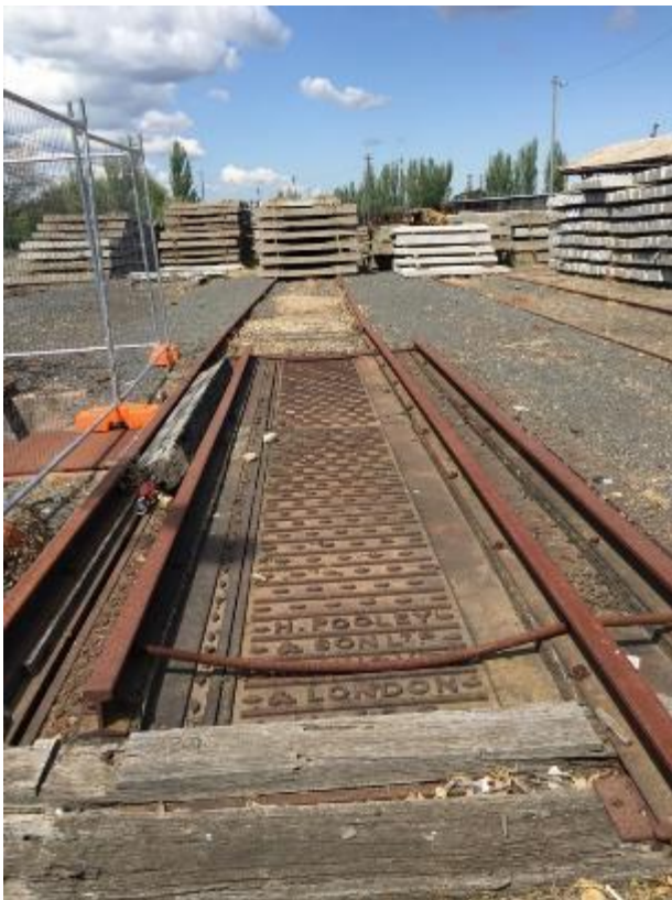
Figure 19 Weighbridge scales
