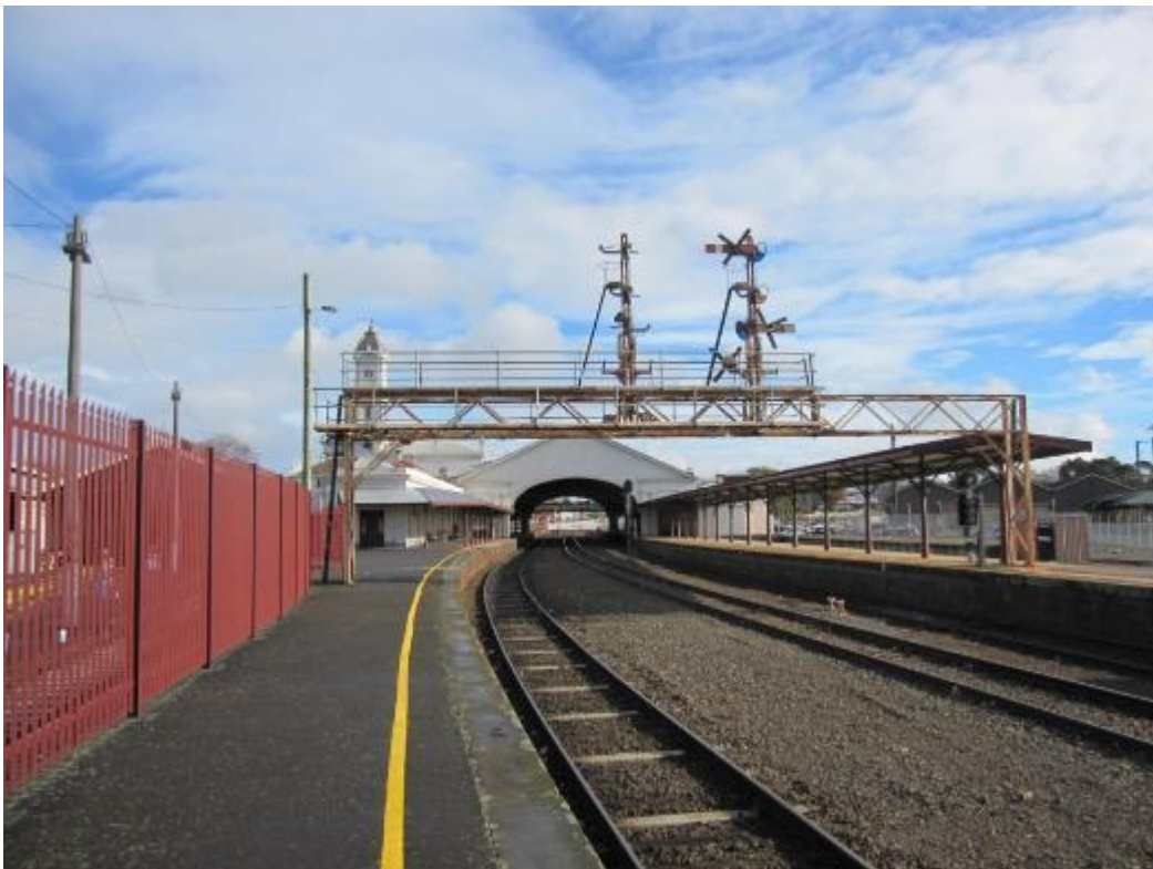
Figure 44 Signal gantries, looking west
