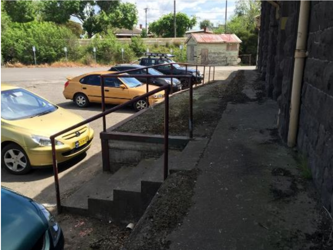
Figure 13 West end of platform to south elevation
