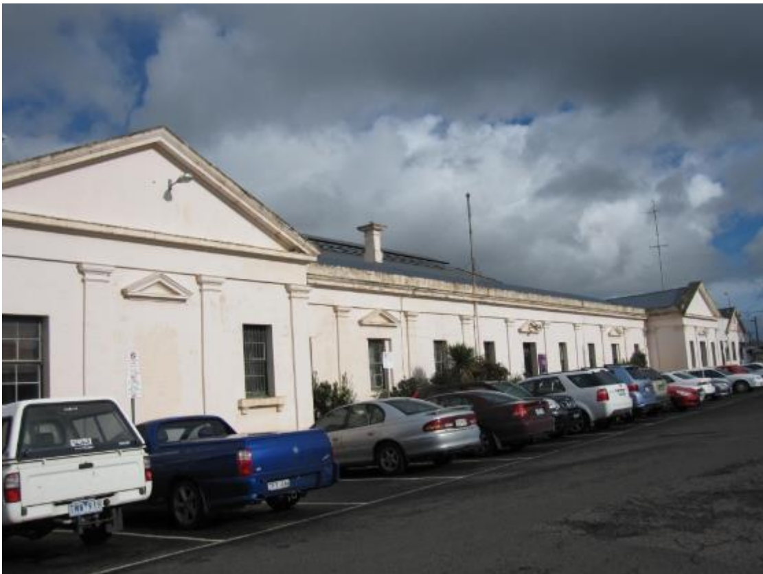
Figure 34 North station building
