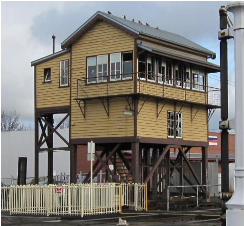
Figure 38 Signal box B
