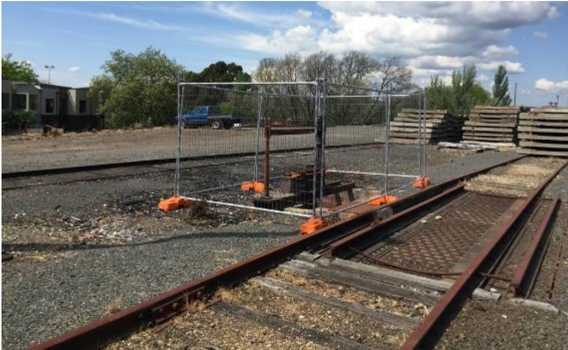
Figure 18 Weighbridge, with fenced equipment at left formerly located within the timber office hut (demolished), and weighbridge scales at right
