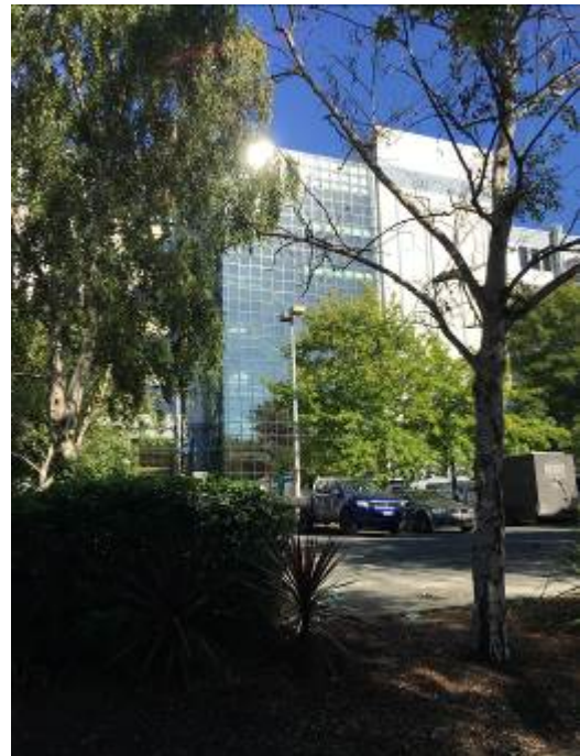
2017: View from corner of Napier Street and Victoria Parade, looking north-west. The glass enclosed staircase is in the centre of the image.
