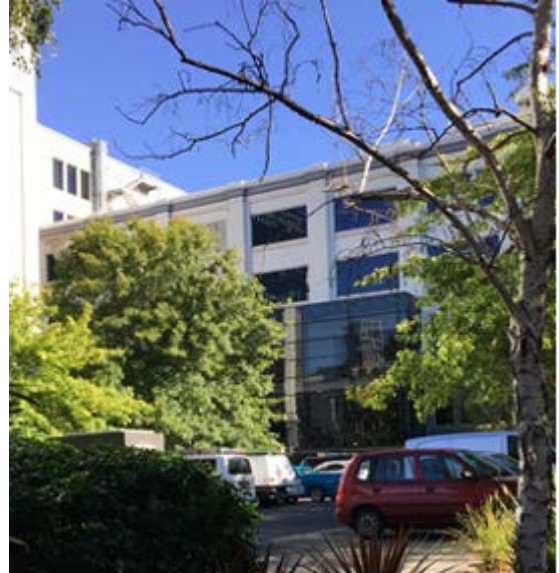
2017: 1931 addition, fronting Victoria Parade. The enclosed glass addition is evident in the centre of the image.
