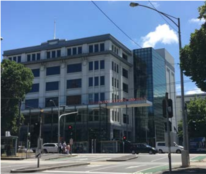
2017: 1924 building, fronting Victoria Parade. The enclosed staircase is evident to the right of the image.
