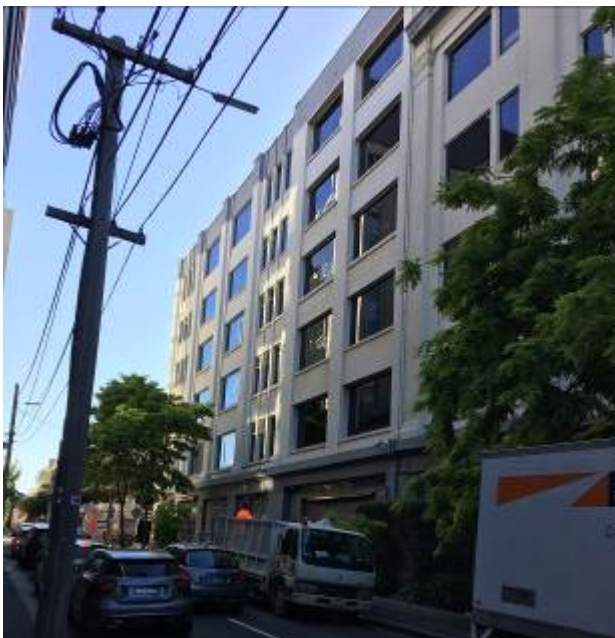
2017: Western elevation. The 10 plate glass windows in the centre of the image indicate the position of the former junction between the 1924 building and the 1931 building, which has been filled in.
