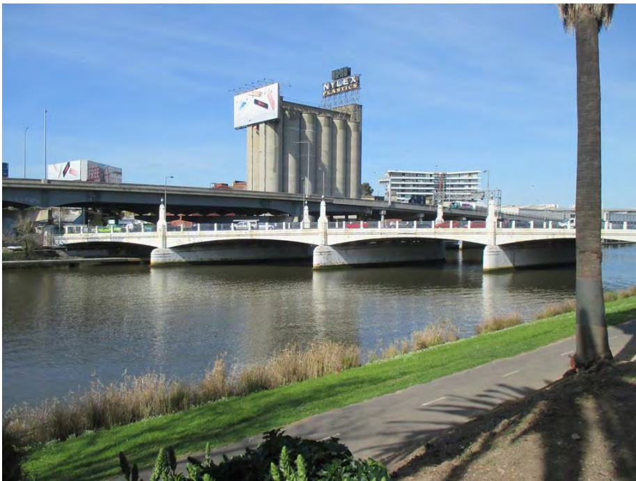
Figure 42 The B9 silos as viewed from Alexandra Avenue looking north-east
