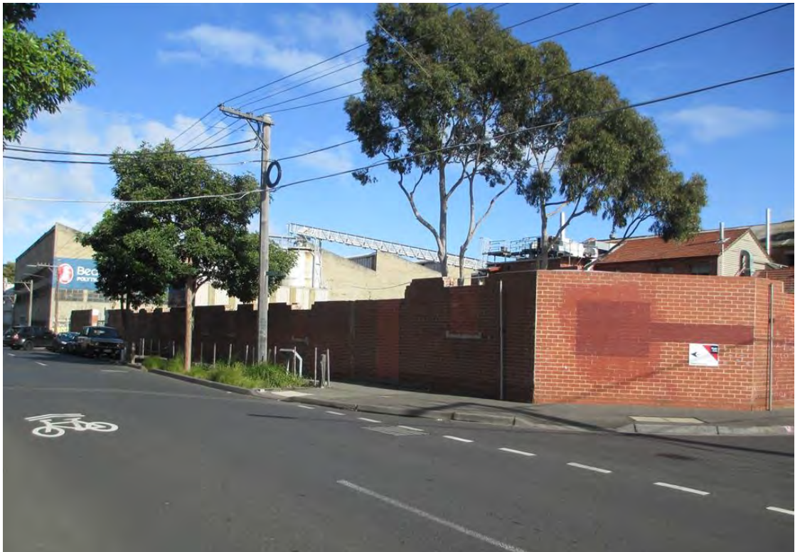
Figure 8 Corner of Gough and Cremorne streets, with wall B1 at the left, and portion of B2 at the right.
