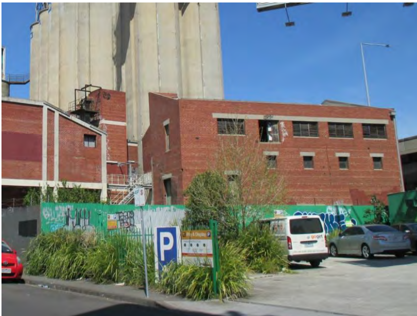
Figure 48 West elevation of B11 (at right); B10 is at left
