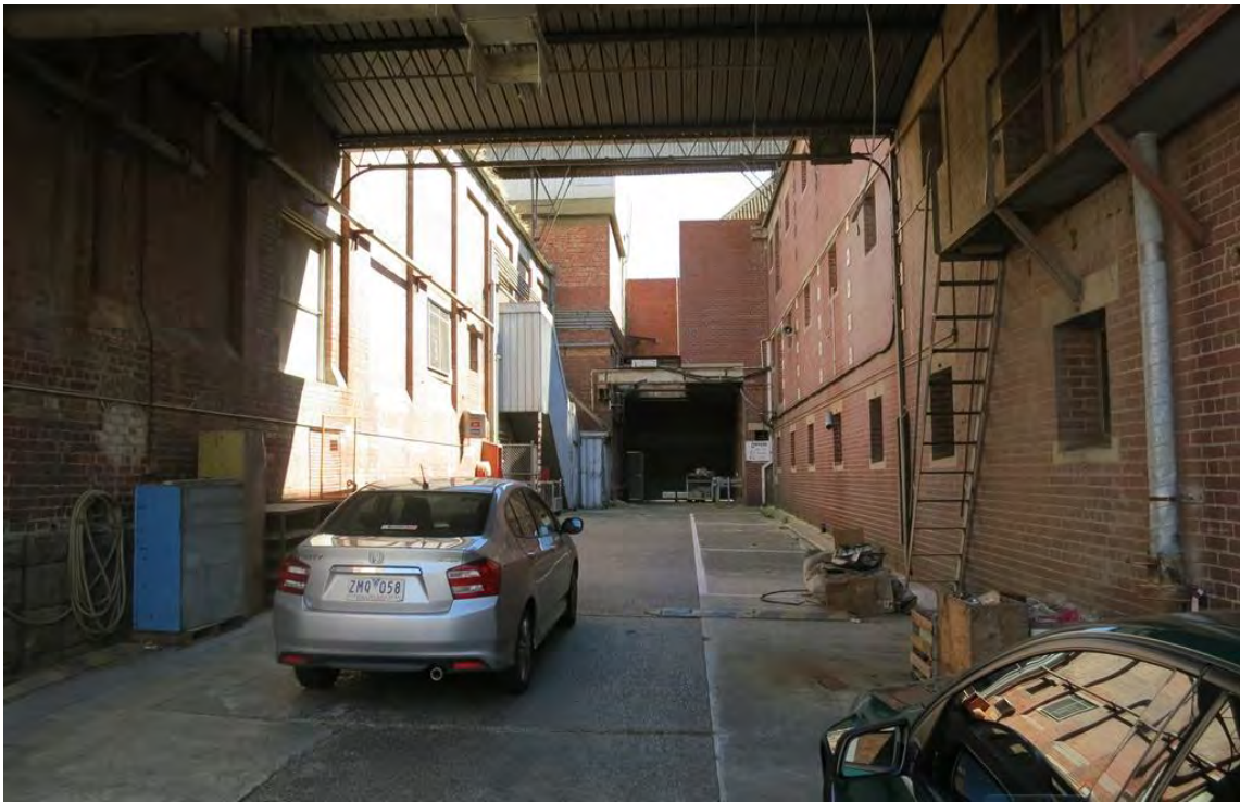
Figure 16 Laneway on north of site, with B4 at right and B5 at left
