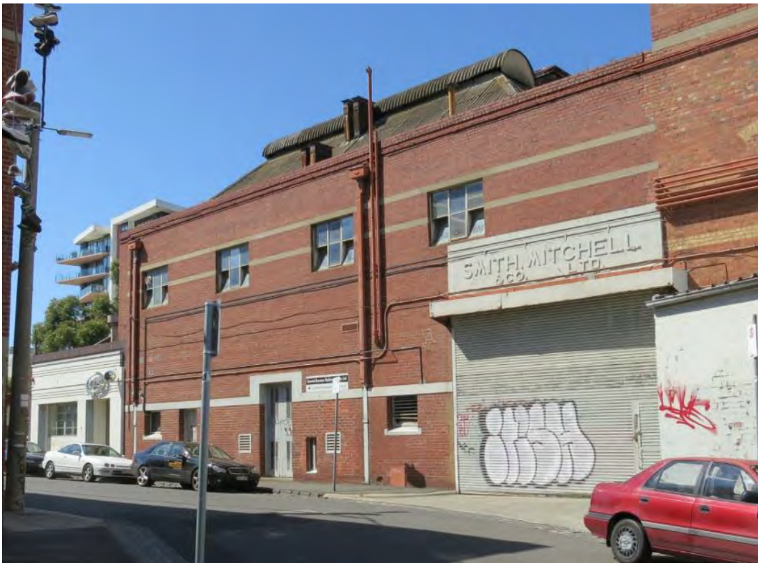
Figure 14 B4, north elevation to Gough Street; the majority of this current form and appearance of the façade will be maintained, as will the barrel vaulted ridge vent to the roof
