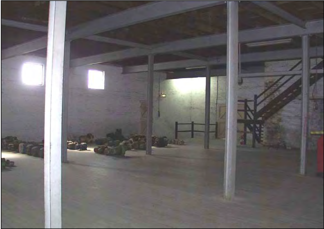
Figure 50 B11, interior of level 1 (middle level)
