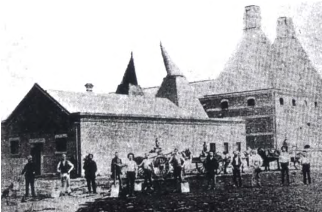
Figure 25 Richmond Maltings, as seen from the east on Cremorne Street, 1881; the (then new) 1880 malt house (B5), with its original kiln roof form, is at right Source: Australian Brewer's Journal . 20 January 1919
