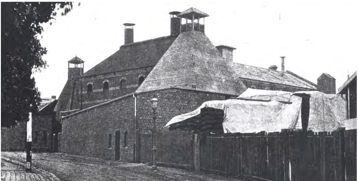
Figure 27 1919 view of Richmond Maltings, on Cremorne Street, showing B5 with the (then new) 1918/19 addition in the foreground Source: Australian Brewer's Journal . 20 January 1919
