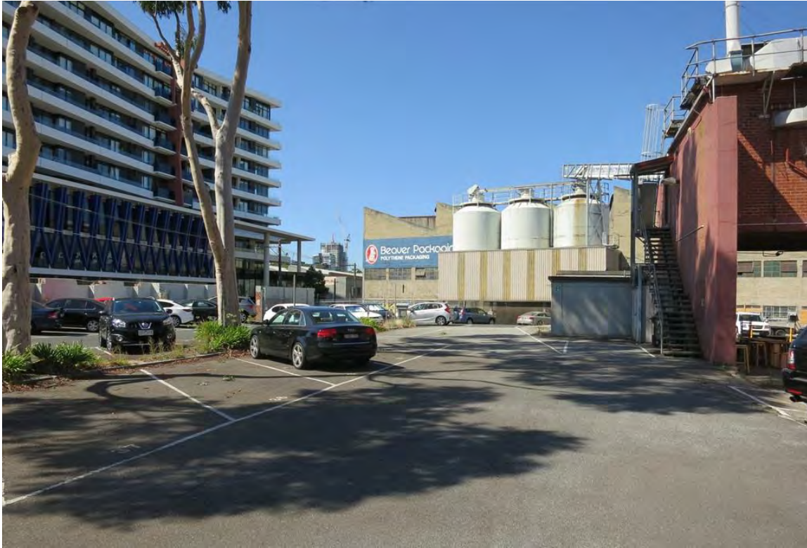
Figure 11 Internal view of east end of site, looking south towards the bulk loading silos
