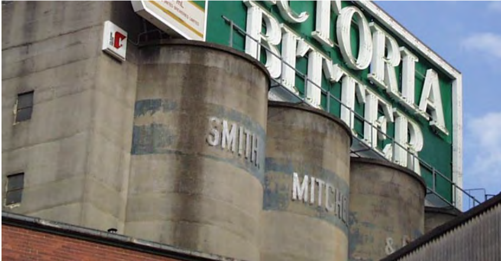
Figure 39 Detail of signage on west side of B8
