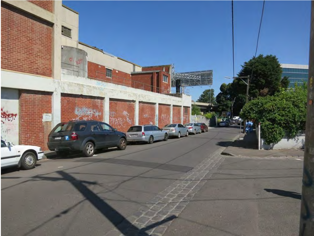
Figure 47 The Gough Street frontage of B10
