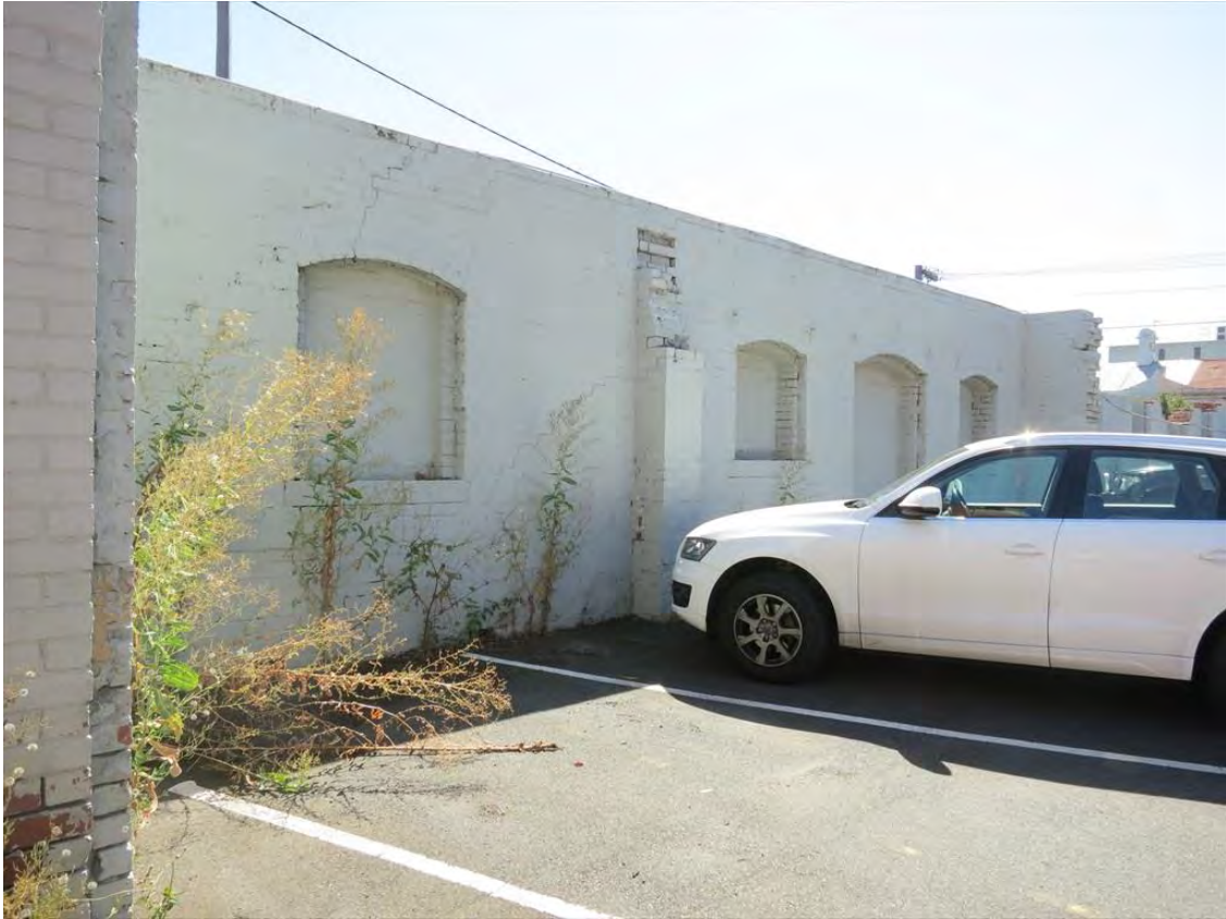
Figure 9 Internal view of wall B2 to Gough Street
