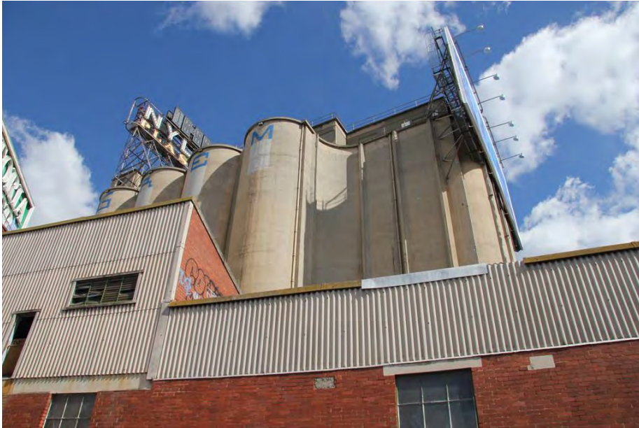
Figure 41 B9 silos, viewed from the north
