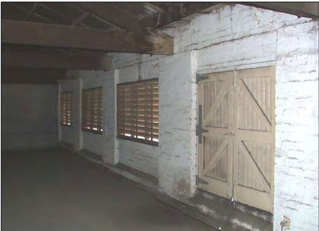
Figure 51 B11, interior of level 2 (top level)
