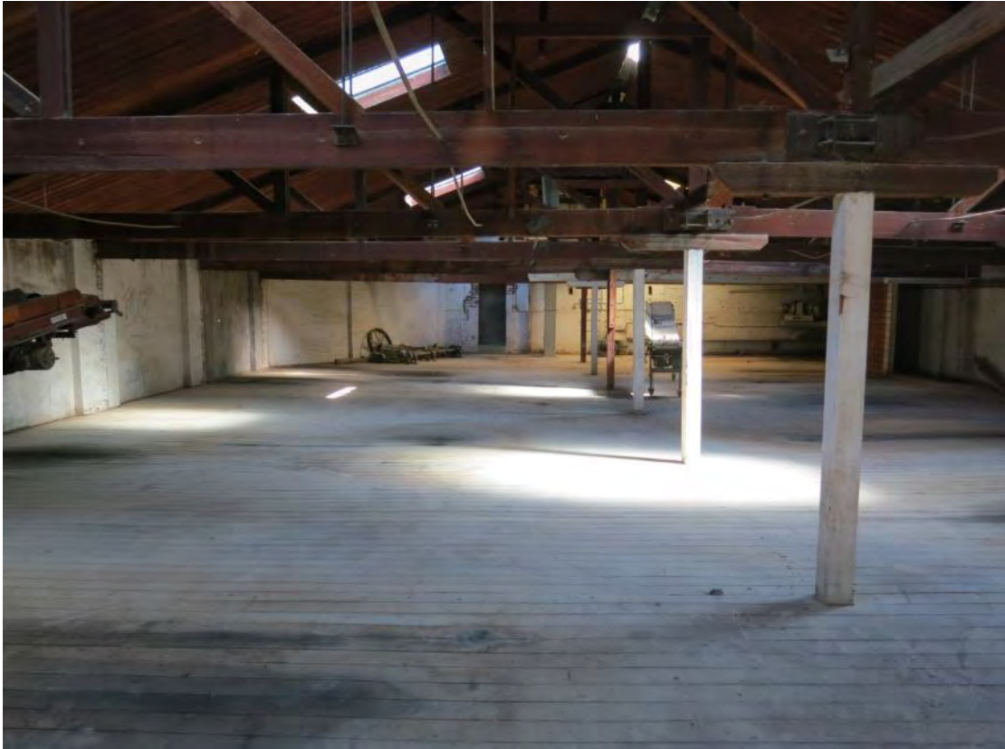
Figure 34 B6 interior, first floor
