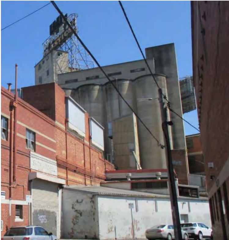
Figure 37 East side of B8 silos, showing concrete cylinders and associated grain elevator tower at right
