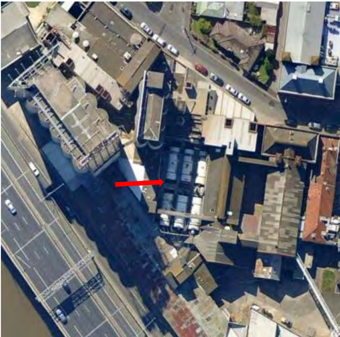
Figure 35 Recent aerial image of the Richmond Maltings site; the location of B7 and the drums, without the roof to the building, is indicated Source: Nearmap
