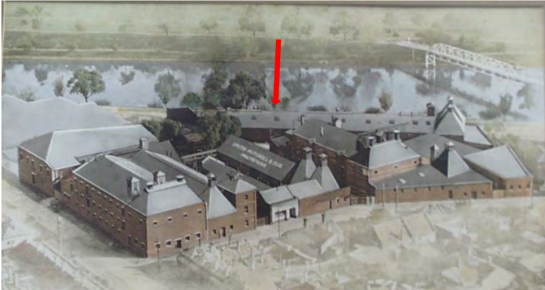
Figure 28 Engraving of Richmond Maltings, late 1920s; the long linear form of B6, the 1920s floor malt house, is in the background adjacent to the Yarra River (indicated by red arrow), prior to the c. 1928 east addition and when it retained its kiln roof forms at the west end; the majority of buildings in the left half of this image were subsequently demolished and/or replaced
