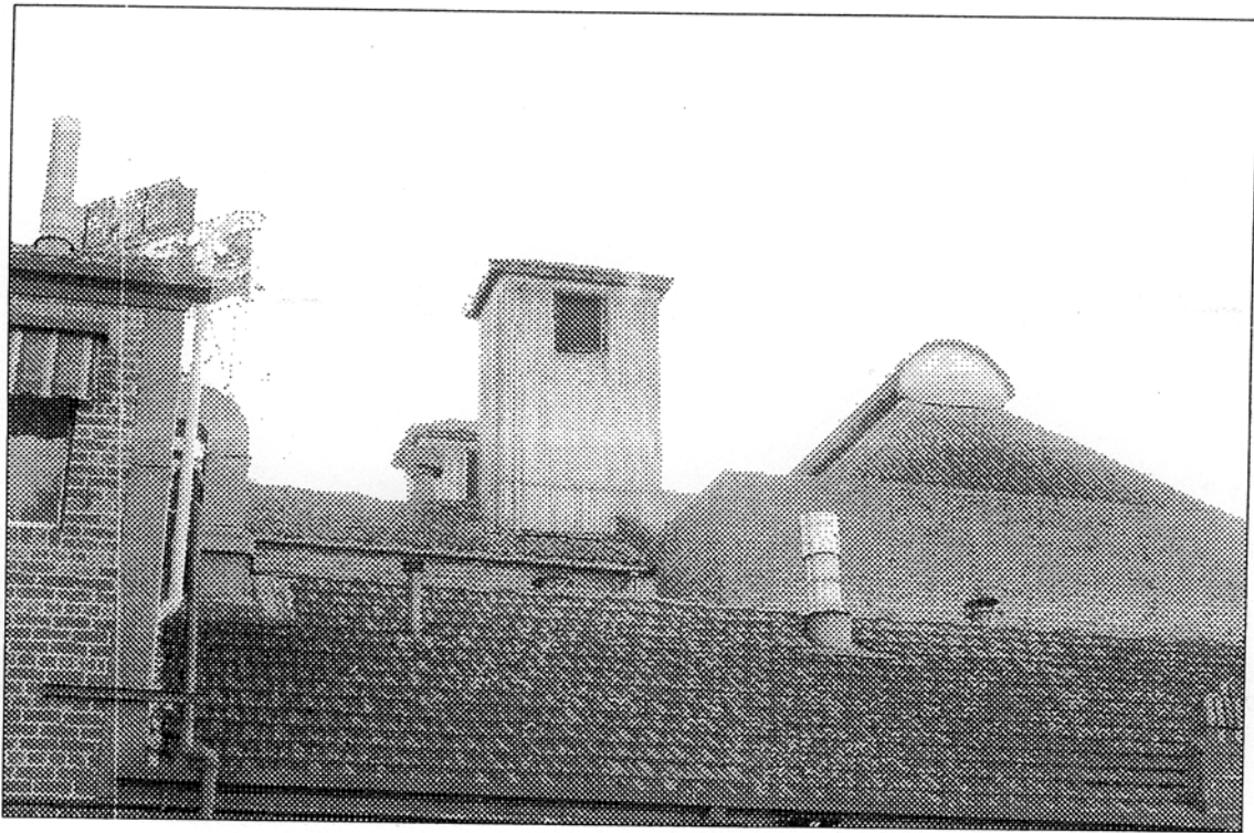
Malthouse Roofline, south side of Gough Street
