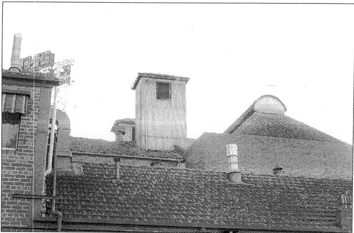
Malthouse Roofline, south side of Gough Street
