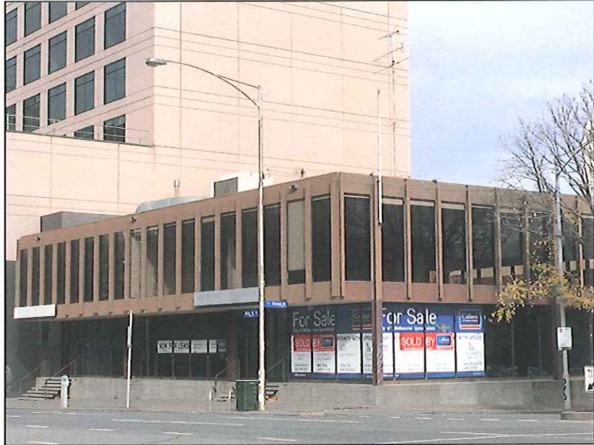
Figure 8 View of the north-east corner of the building with the brown external treatment visible and some of the rooftop plant.
