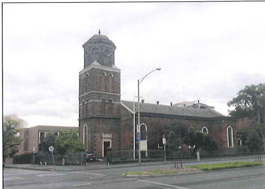
Figure 13 View of St James Old Cathedral from the diagonally opposite side of King Street.
