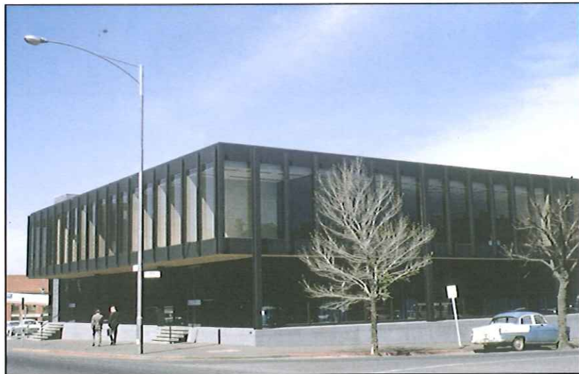
Figure 1 A c.1970 photograph of the newly completed offices of Yuncken Freeman architects showing the steelwork painted black or similarly dark colour. Source: State Library of Victoria.
