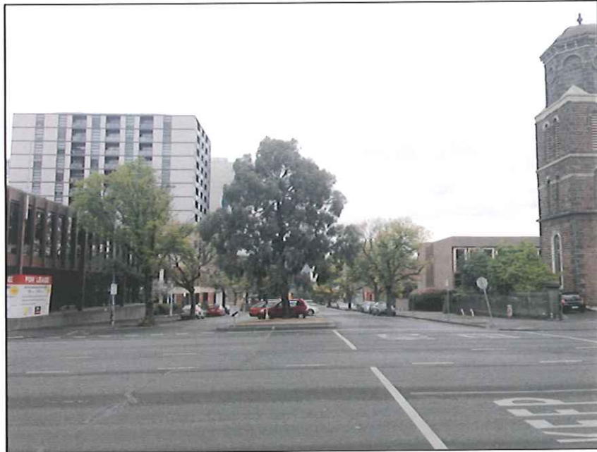
Figure 16 View west along Batman Street from the opposite (east) side of the intersection with King Street. The subject site is visible to the left.
