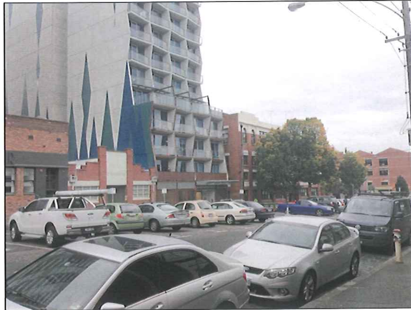
Figure 12 View along the south side of Batman Street to the south-west, showing the recently constructed apartment tower at 49 Batman Street centre left, next to the former Keep Bros. & Wood factory at 55 Batman Street (centre right).
