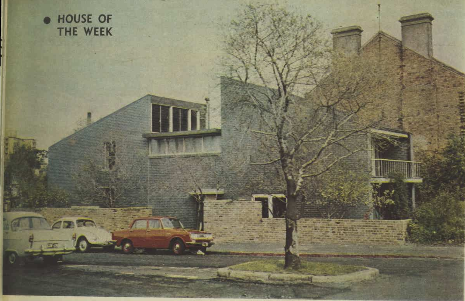
Old bricks were used for the high fence which gives privacy to two tiny courtyards. Only breaks with convention on the outside of the house are the side entrance instead of a front one and the interruption in the sloped slate roof, which allows for extra windows.
