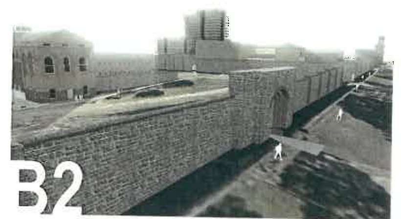
view B2 taken from RL 70.89 (existing RL adjacent to roller door is 61.74) and the target RL is set at 32.49
